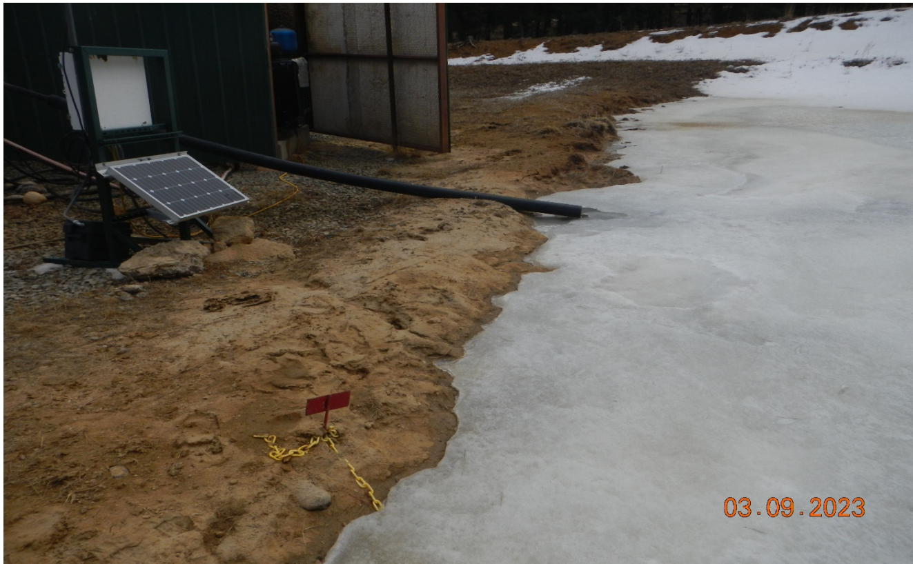
Photo 2. The water level is above 2 ft. freeboard.
