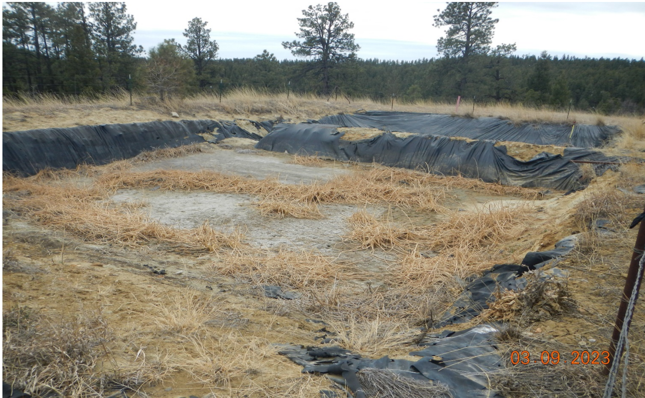
Photo 6. Facing southeast toward the pit. The pit liner is torn and degraded.
