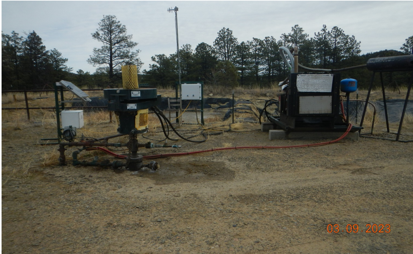
Photo 4. Facing toward the wellhead. There is a slight water leak at wellhead.
