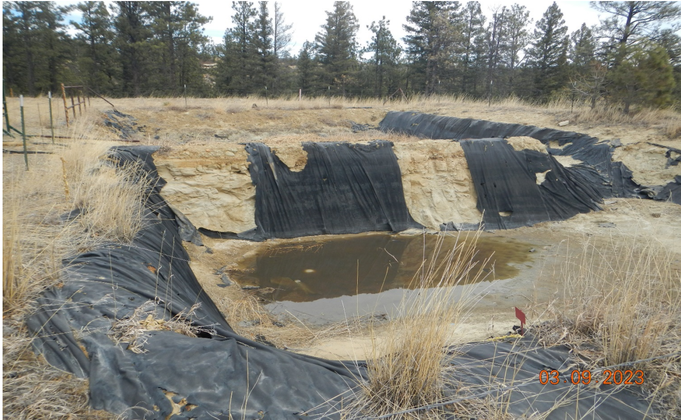
Photo 5. Facing northeast toward the pit. The pit liner is torn and degraded.
