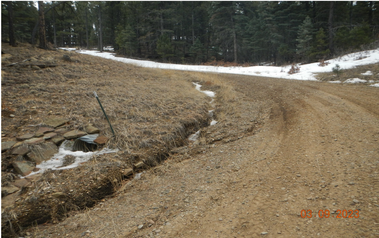
Photo 1. Facing toward the switch back of the access road. There is erosion beginning to occur in this area which should be addressed.
