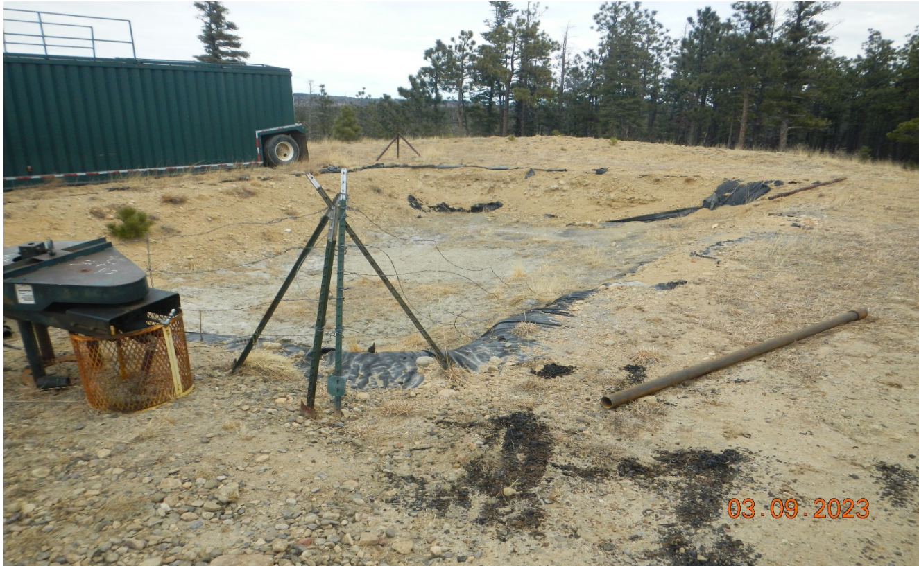
Photo 4. The pit liner and fence are degraded and not maintained.
