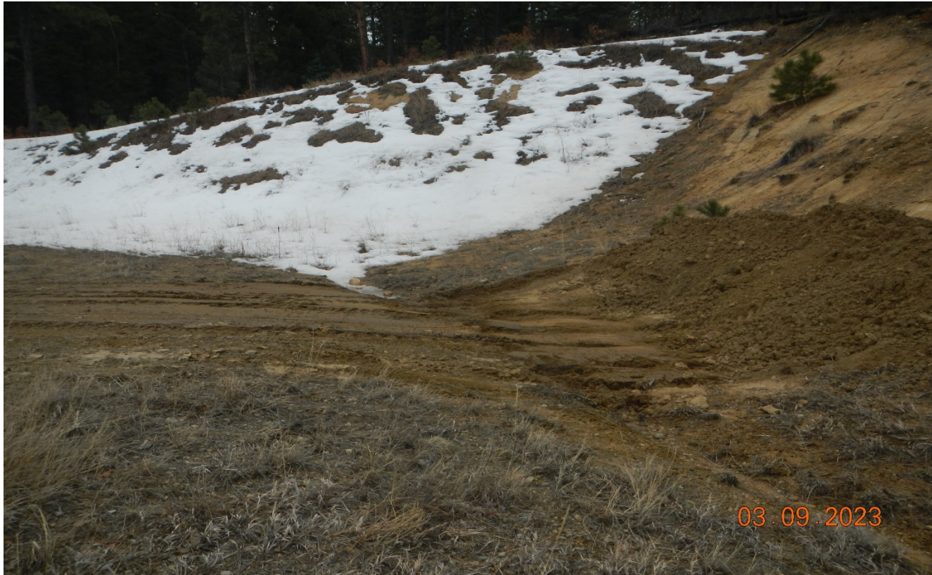
Photo 7. Facing toward the southwest cut slope. Soils were pushed out to allow better drainage however loose soils pushed out need to be stabilized.
