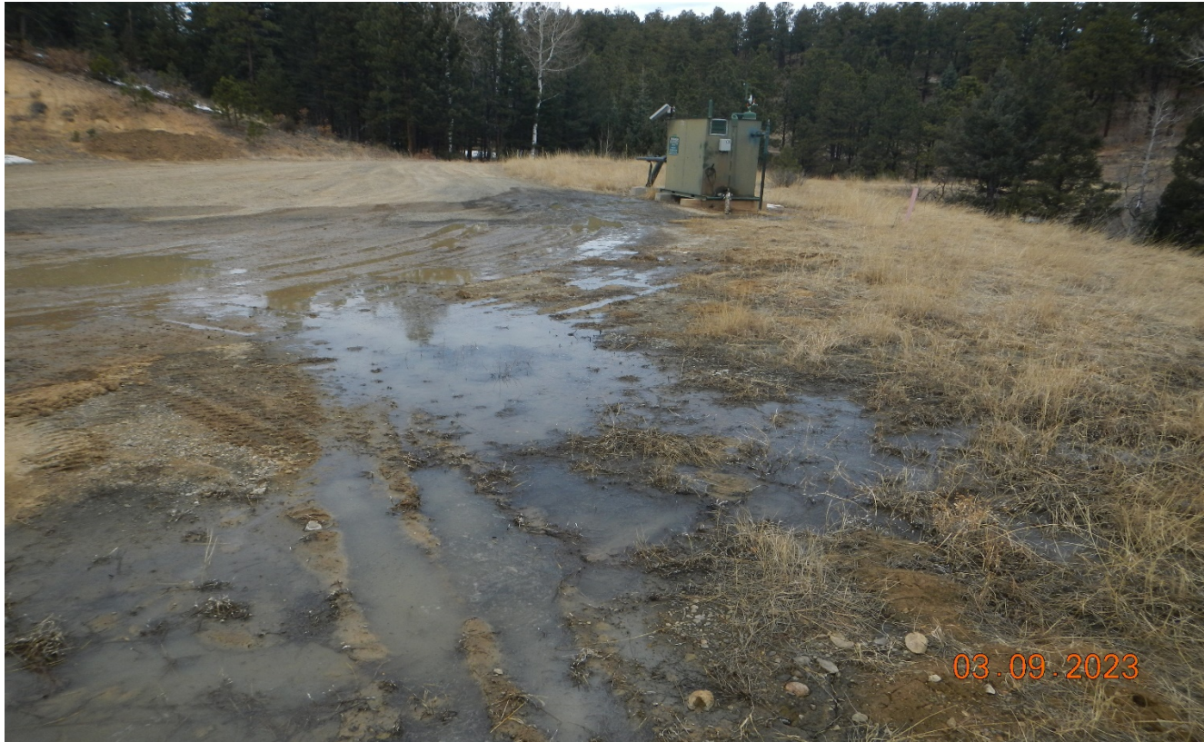
Photo 5. Facing northwest at the location showing spread of water leak across the location.
