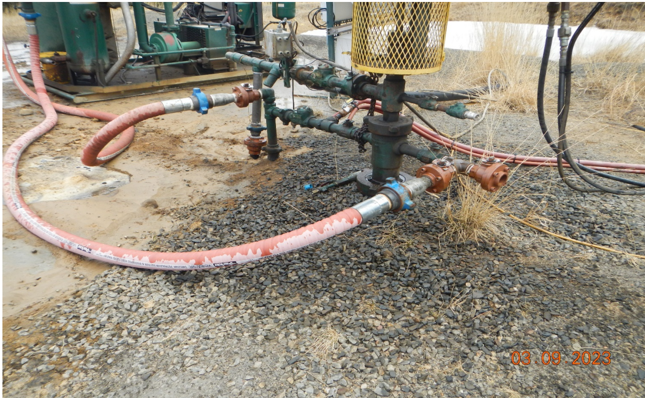
Photo 3. There is stained soil around the wellhead that needs to be cleaned up.
