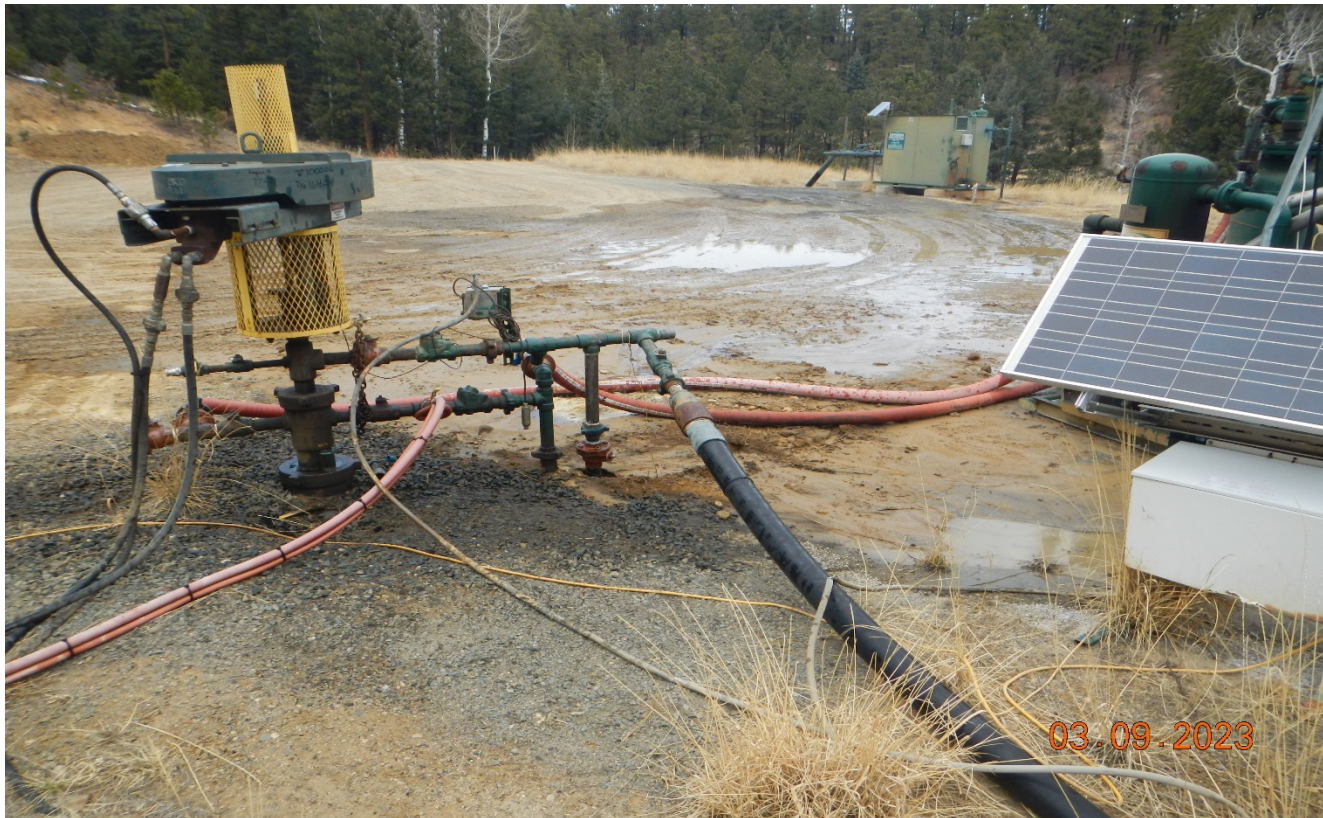
Photo 4. The water leak is flowing across the location toward the meter shed.
