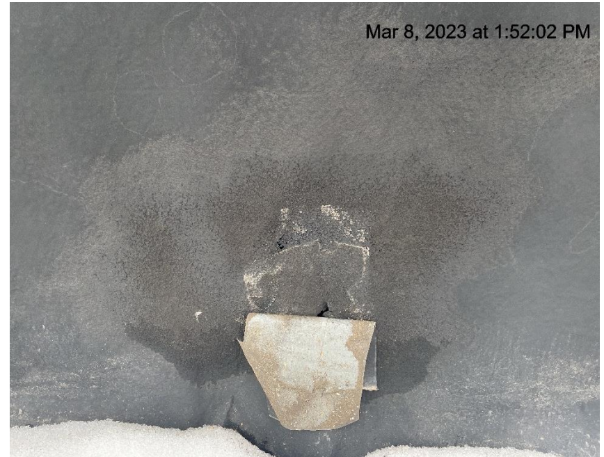
Photo # 1995 Containment liner needs maintenance
