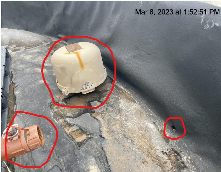
Photo # 1997 Open ended load line, unused equipment & hole in containment liner
