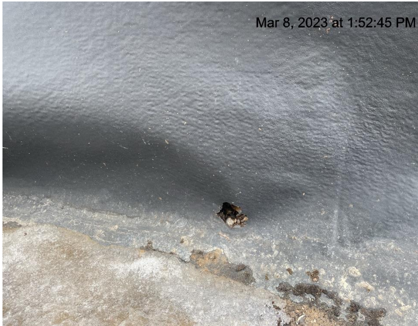
Photo # 1996 Containment liner needs maintenance
