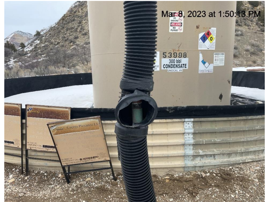
Photo # 1992 Flowline heating insulation open ended
