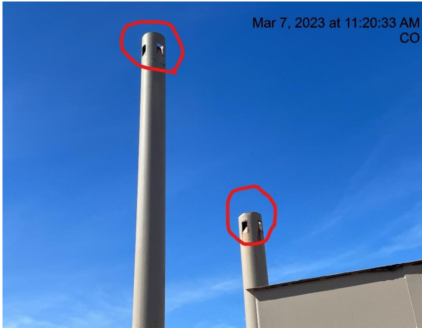
Photo # 1771 Bird protectors missing
