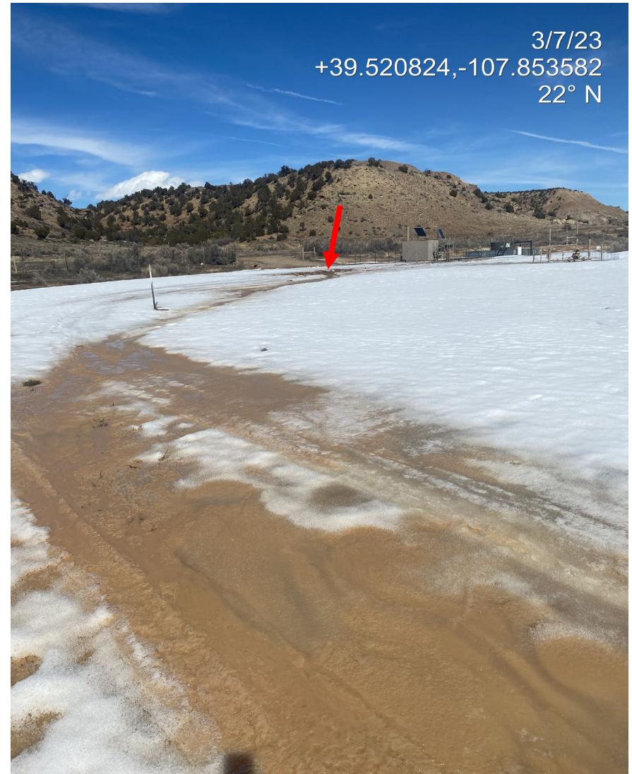
Photo 4. Photos show degradation to the pad surface. Degraded pad is acting as a sediment source. Note sediment laden stormwater within ruts (left) and sediment from degraded pad flowing off location (right). Arrow indicates area of ruts shown in left photo.
