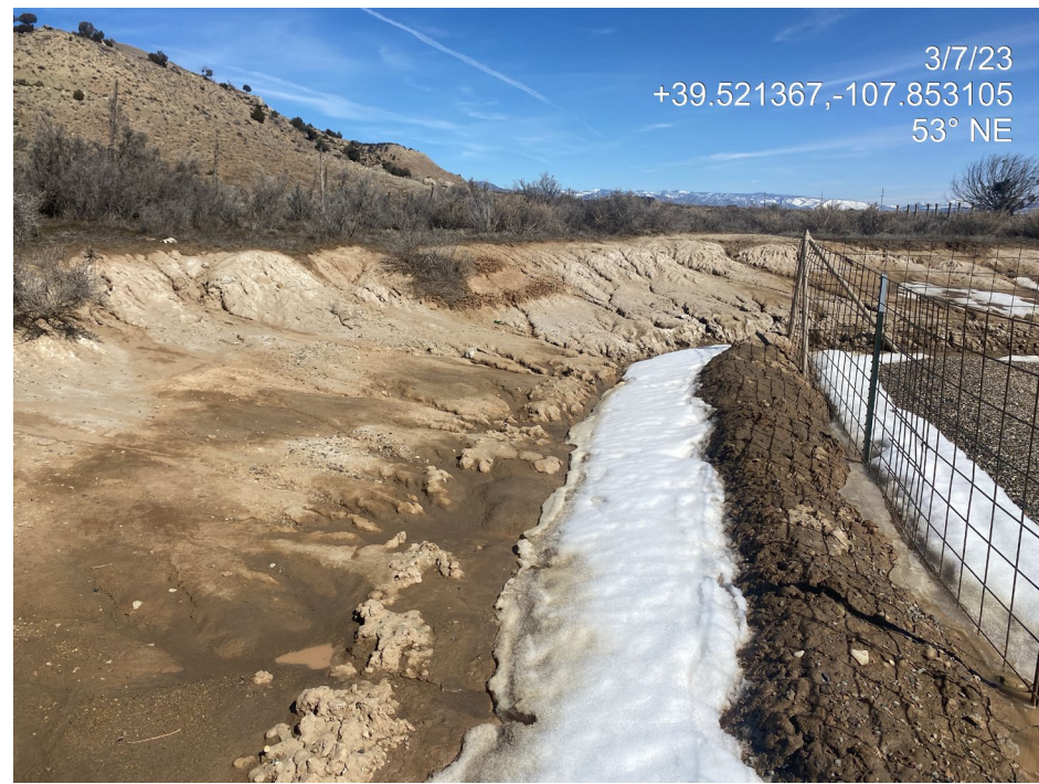
Photo 3. Photos show erosion degradation occurring on the slope at the northeast of the location. Slopes are bare and unprotected.
