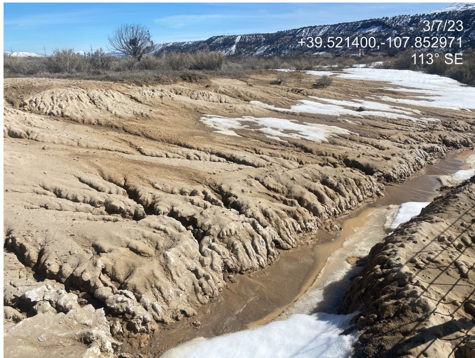
Photo 3. Photos show erosion degradation occurring on the slope at the northeast of the location. Slopes are bare and unprotected.
