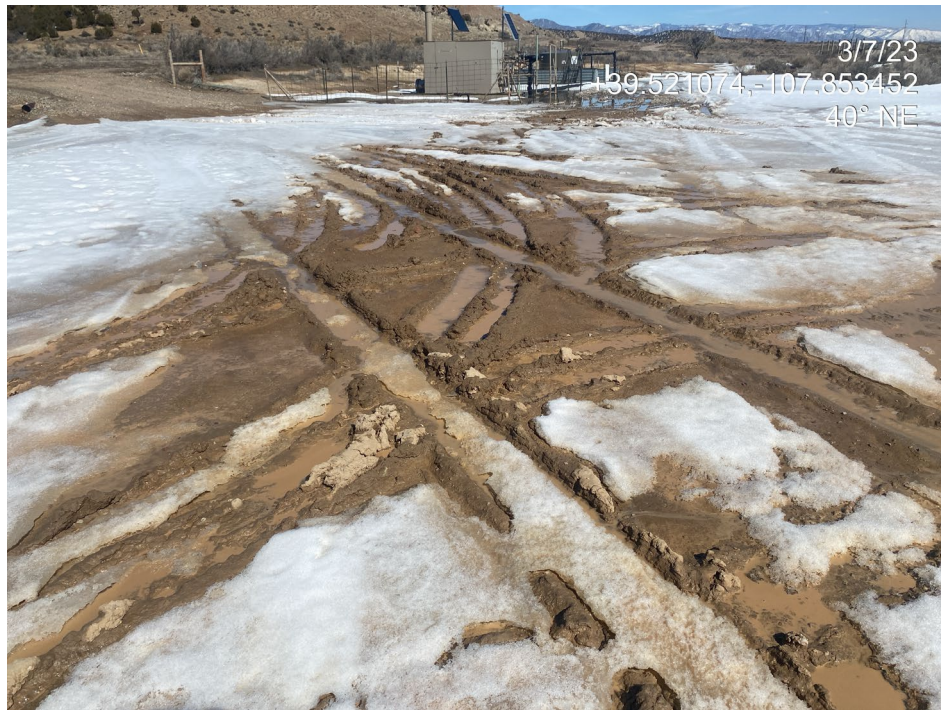
Photo 4. Photos show degradation to the pad surface. Degraded pad is acting as a sediment source. Note sediment laden stormwater within ruts (left) and sediment from degraded pad flowing off location (right). Arrow indicates area of ruts shown in left photo.
