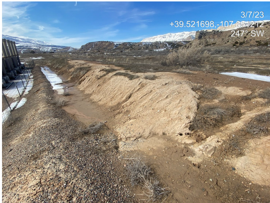
Photo 4. Photos show erosion degradation occurring on the slope to the north of the separators. Slopes are bare and unprotected. Only annual vegetation is present.
