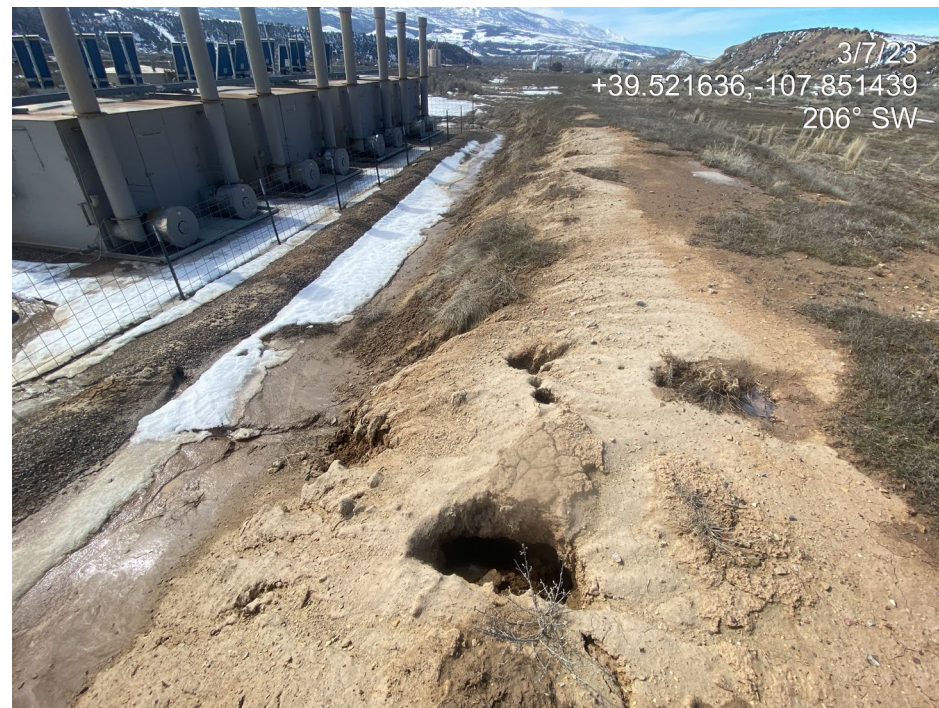
Photo 4. Photos show erosion degradation occurring on the slope to the north of the separators. Slopes are bare and unprotected. Only annual vegetation is present.
