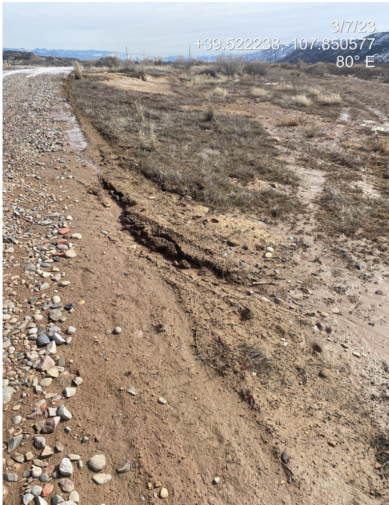
Photo 3. Photos show rill erosion occurring adjacent to the access road.
