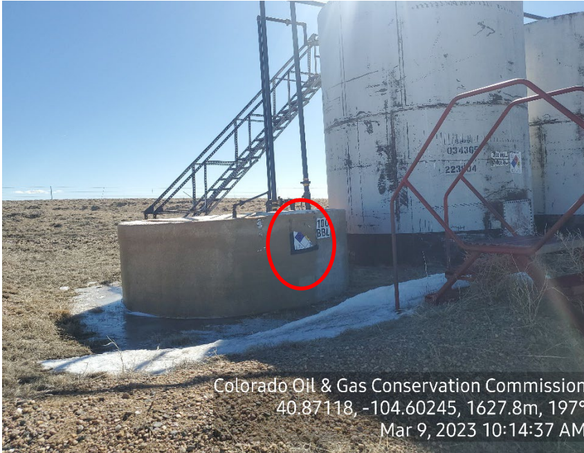
Photo 5: NFPA placarding damaged
