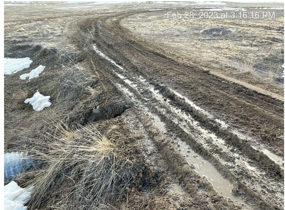
Photo 5. Photo of access road at culvert, sediment laden stormwater leaving site.
