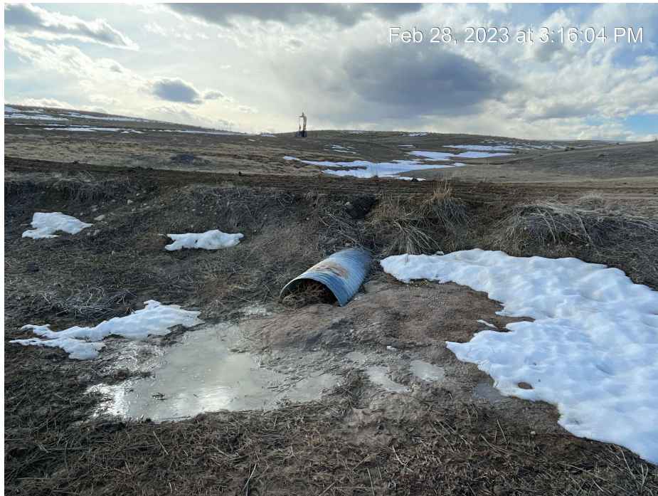
Photo 4. Photo taken of culvert outlet on access road just prior to pad.
