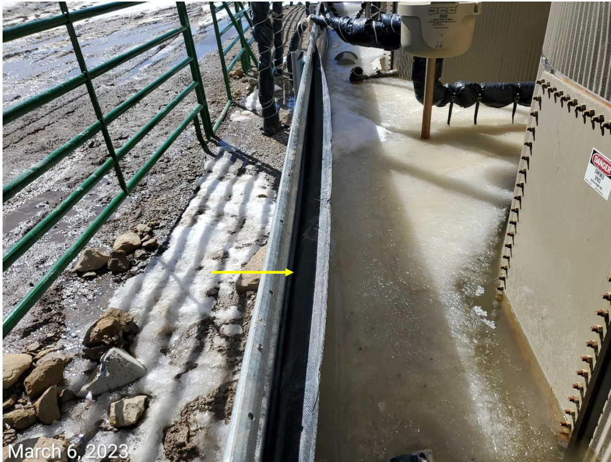
Photo 3: Photo example of areas where liner is separating from the metal containment berm.
