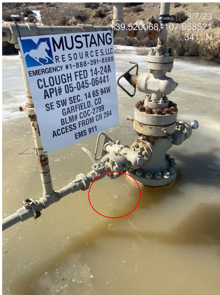
Photo 2. Photos show the area around well API # 045-06441 is inundated with stormwater. Bubbles are rising in the water indicative of a leak.
