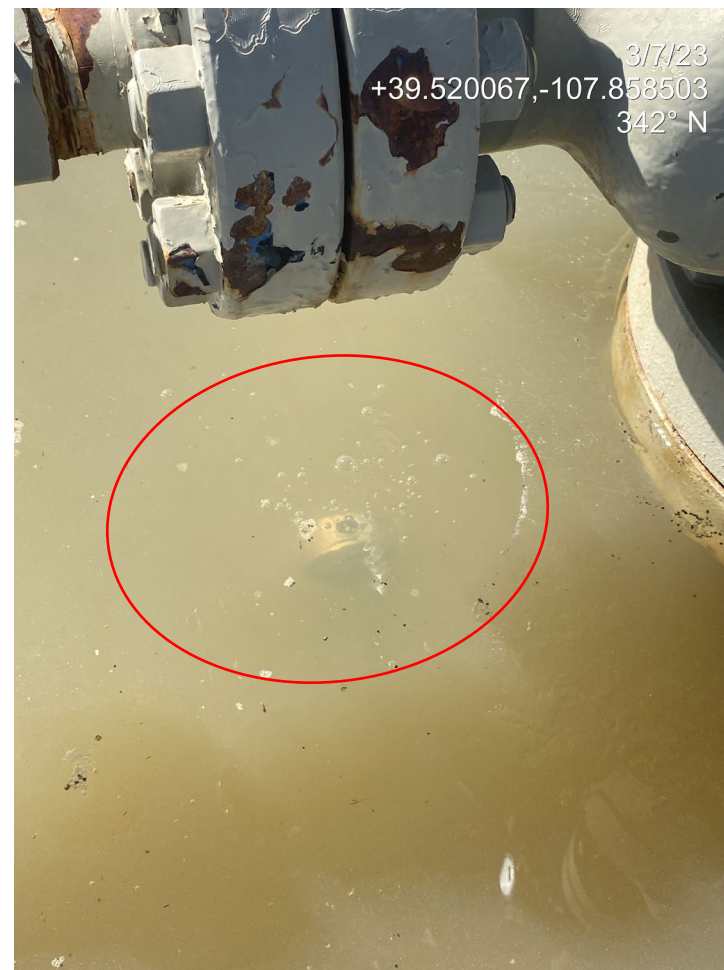
Photo 2. Photos show the area around well API # 045-06441 is inundated with stormwater. Bubbles are rising in the water indicative of a leak.
