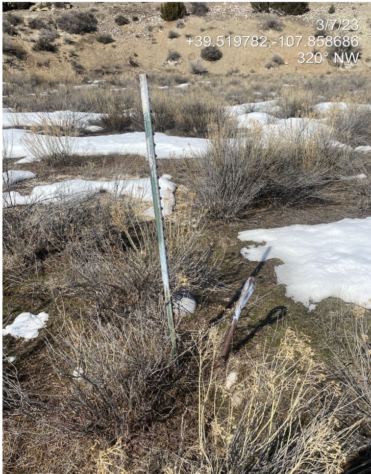
Photo 3. Photos taken from the western interim area (left) and working pad area (right) show examples of anchor markers. All anchor markers on location have faded and are no longer marked with a bright color.
