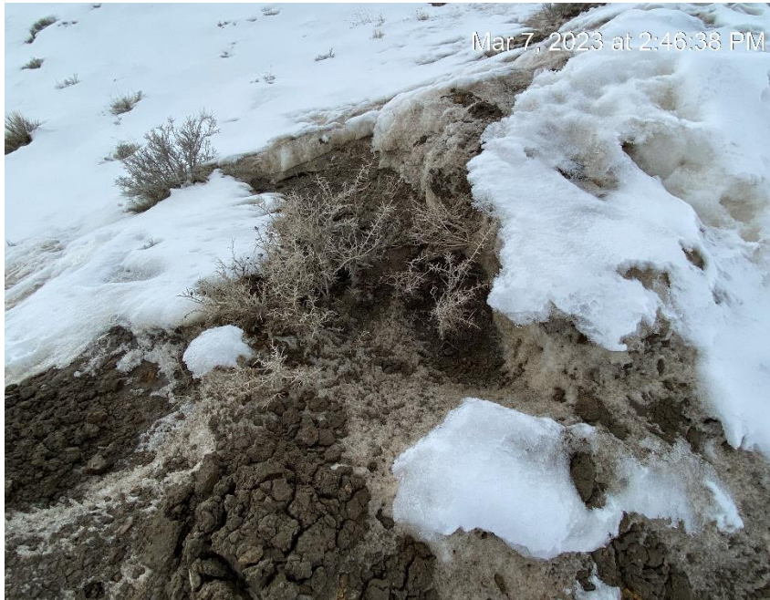
Soil migration from being pushed off location during snow removal
