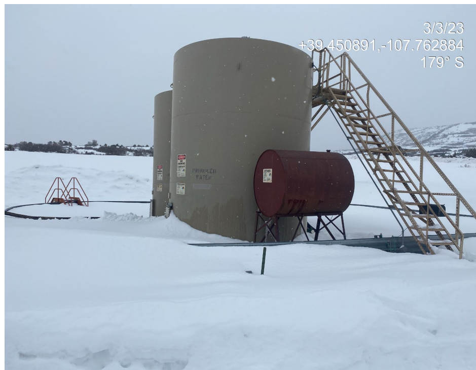
Photo 3. Photos show production areas. Tank battery sign absent at northeastern battery (left).
