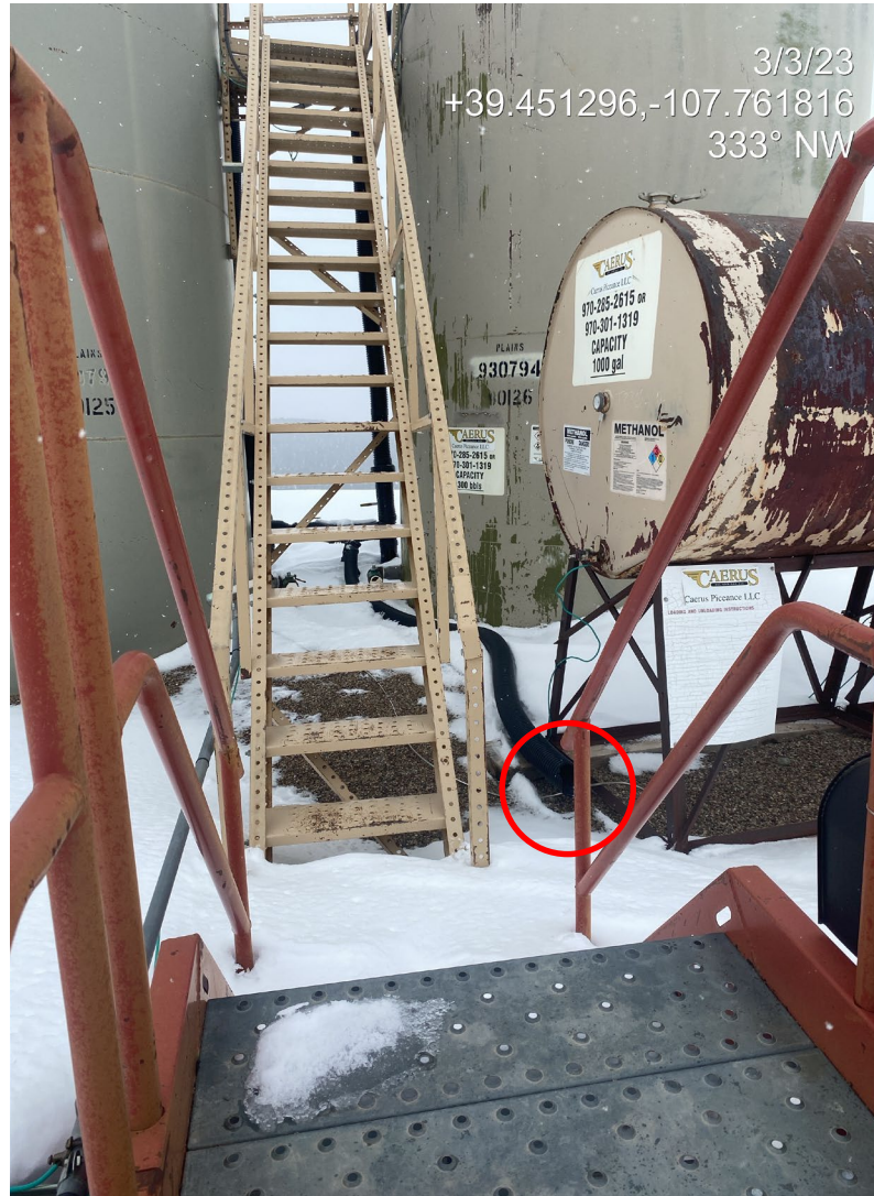
Photo 2. Photo shows piping at the tank battery is open ended/lacks wildlife protection BMPs.
