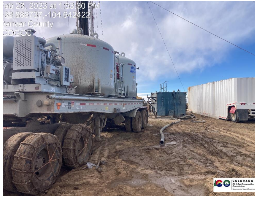
Pic 2 Cement truck/tanks
