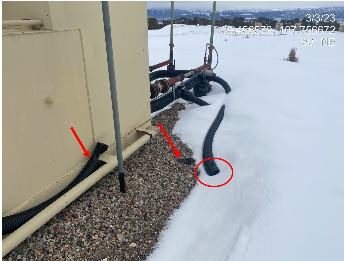
Photo 2. Photo shows wildlife protection BMPs to prevent entry into separator piping are absent (circled). Photo also shows trash (arrows).
