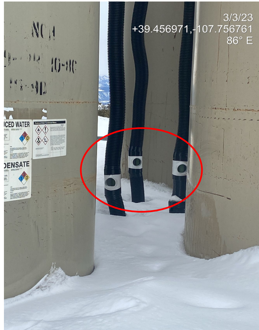
Photo 3. Photo shows wildlife protection BMPs to prevent entry into tank battery piping are absent.
