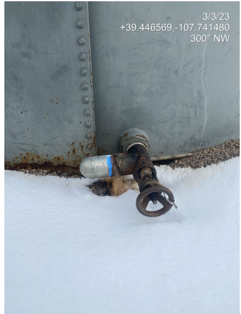
Photo 2. Photos show fluid released from a produced water/condensate tank drain.
