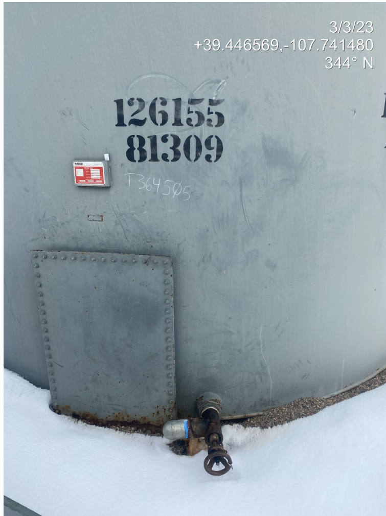
Photo 2. Photos show fluid released from a produced water/condensate tank drain.
