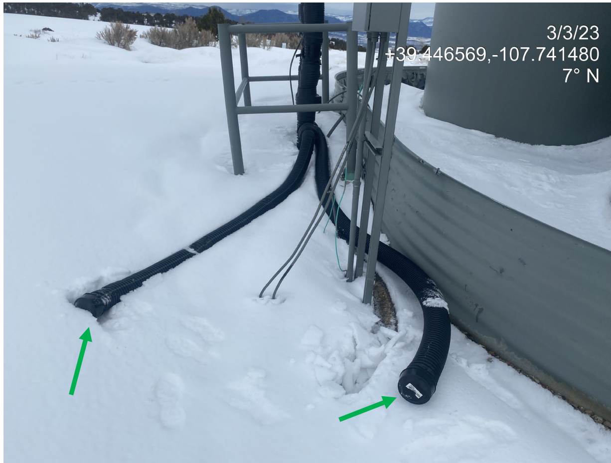
Photo 4. Photo shows caps are installed on piping at the tank battery.
