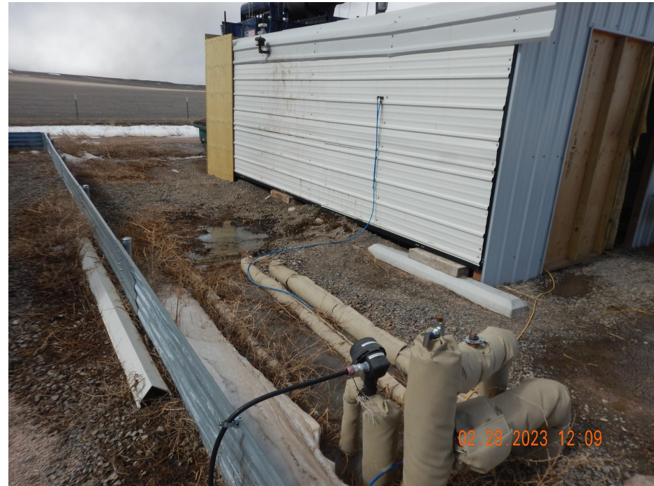
Photo 6. Photo taken from the western location, facing West. Photo illustrates stained soil/spill related to the compressor.
