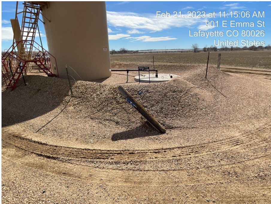
Photo 5. Photo taken of downed perimeter fence of tank battery.
