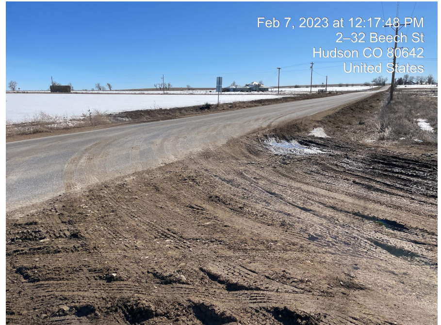
Photo 2. Facing toward county road from location entrance. Evidence of tracking on to the pavement.
