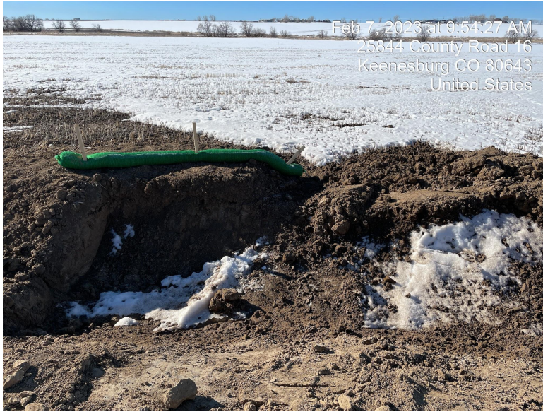
Photo 3. Photo of wattles on Southwest corner sediment trap. Wattle on top of berm not in sediment trap spillway. Wattle needs to be moved to spillway.
