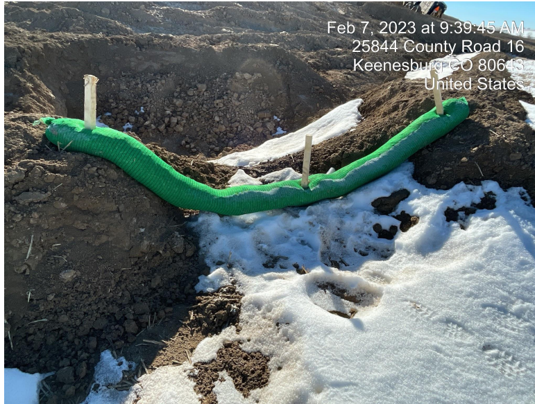
Photo 1. Photo of wattle on Northwest corner sediment trap. Wattle need to be reset.
