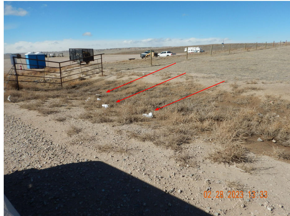
Photo 7. Photo taken from a portion of the access road, facing East. Photo illustrates Operator has conducted snow removal on the access road and is creating additional disturbances by plowing road base onto reference areas.
