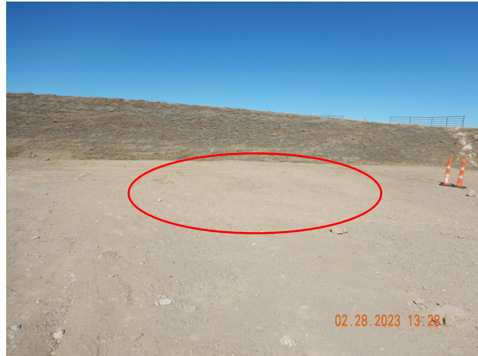
Photo 2. Photo taken from the northeastern location, East. Photo illustrates the pit has been backfilled prior to receiving approval by COGCC.
