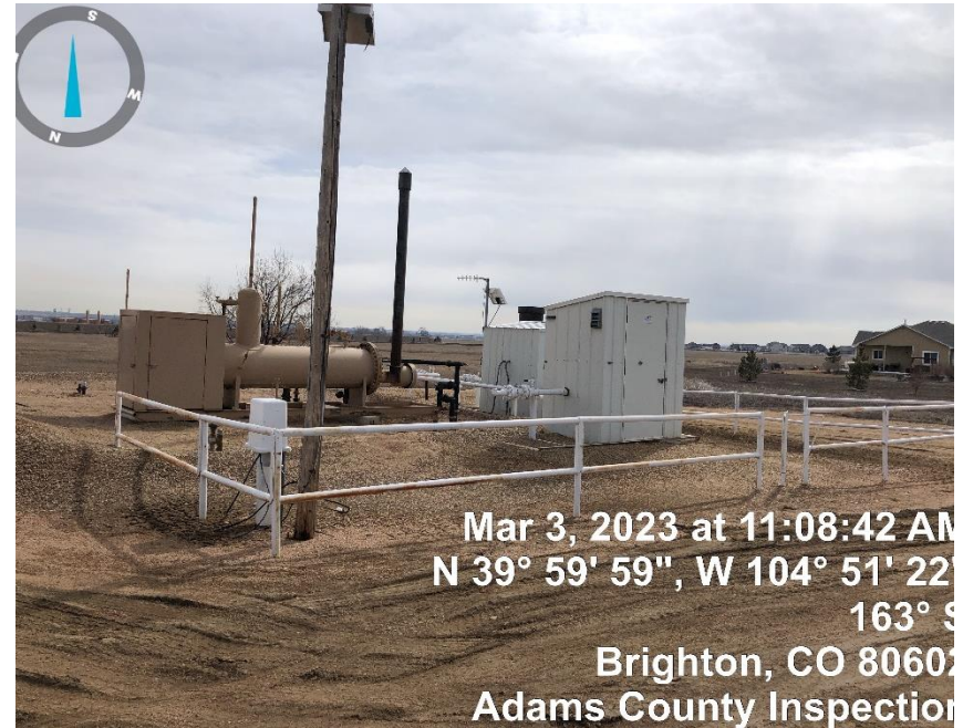
Photo#2 Separator/(2)Gas Meters/ECD/
