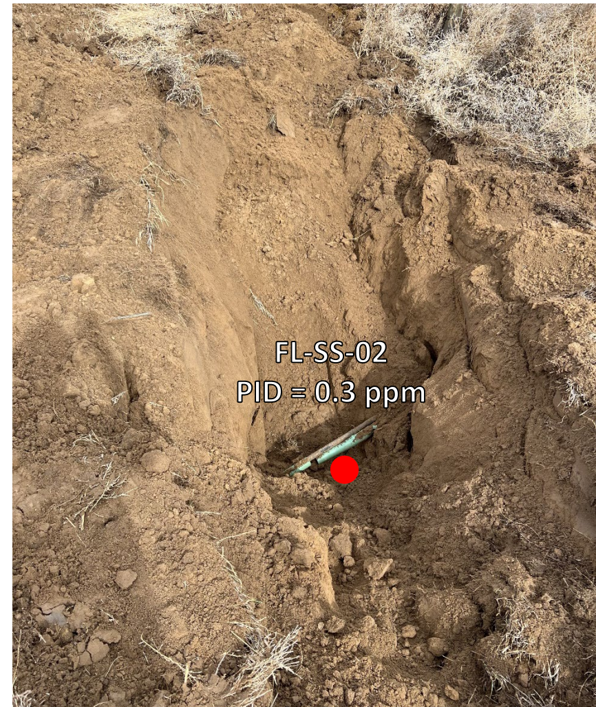
Looking northeast at bellhole/cut point for removal – field screened
