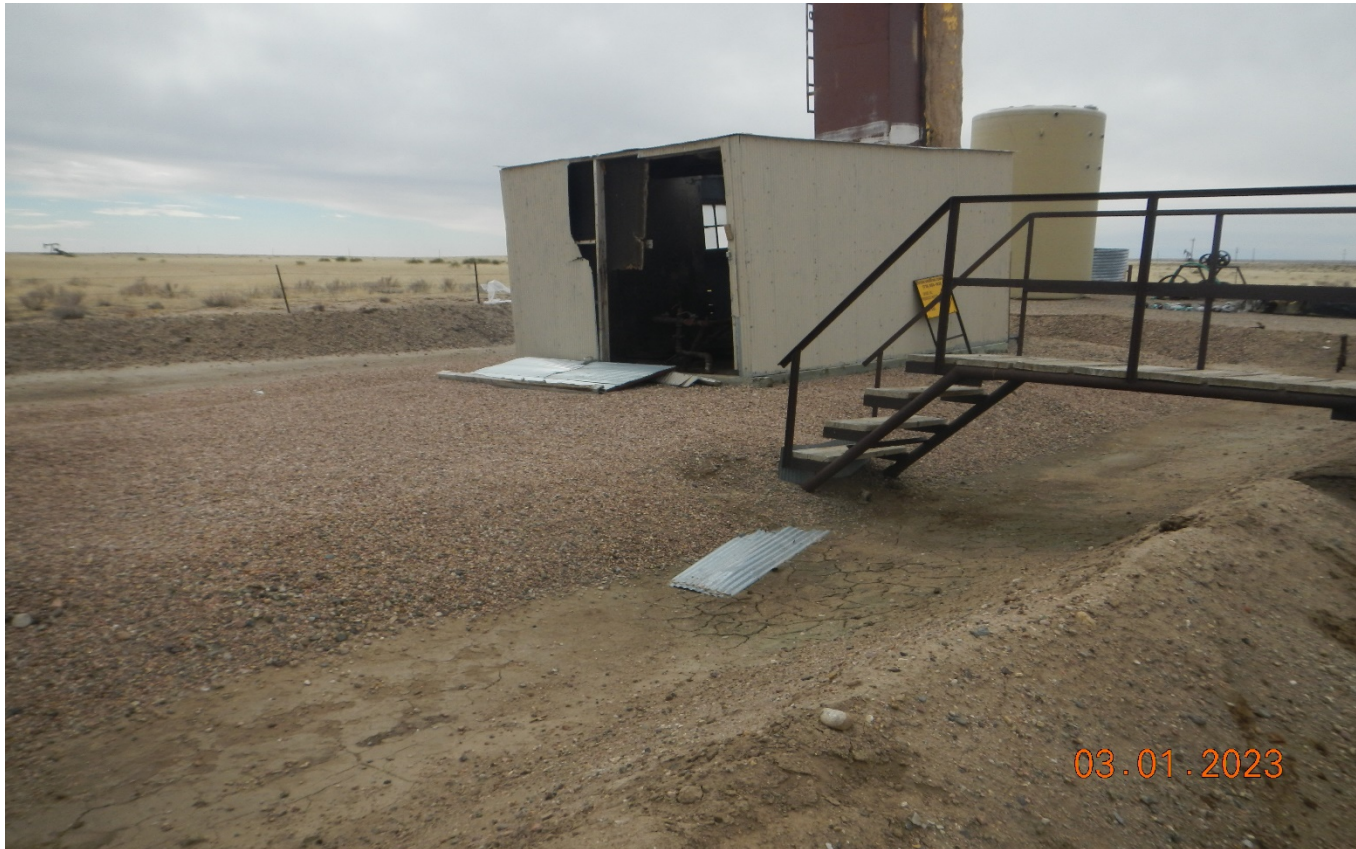
Photo 6. The shed inside the containment battery is not maintained with metal siding laying on the ground.
