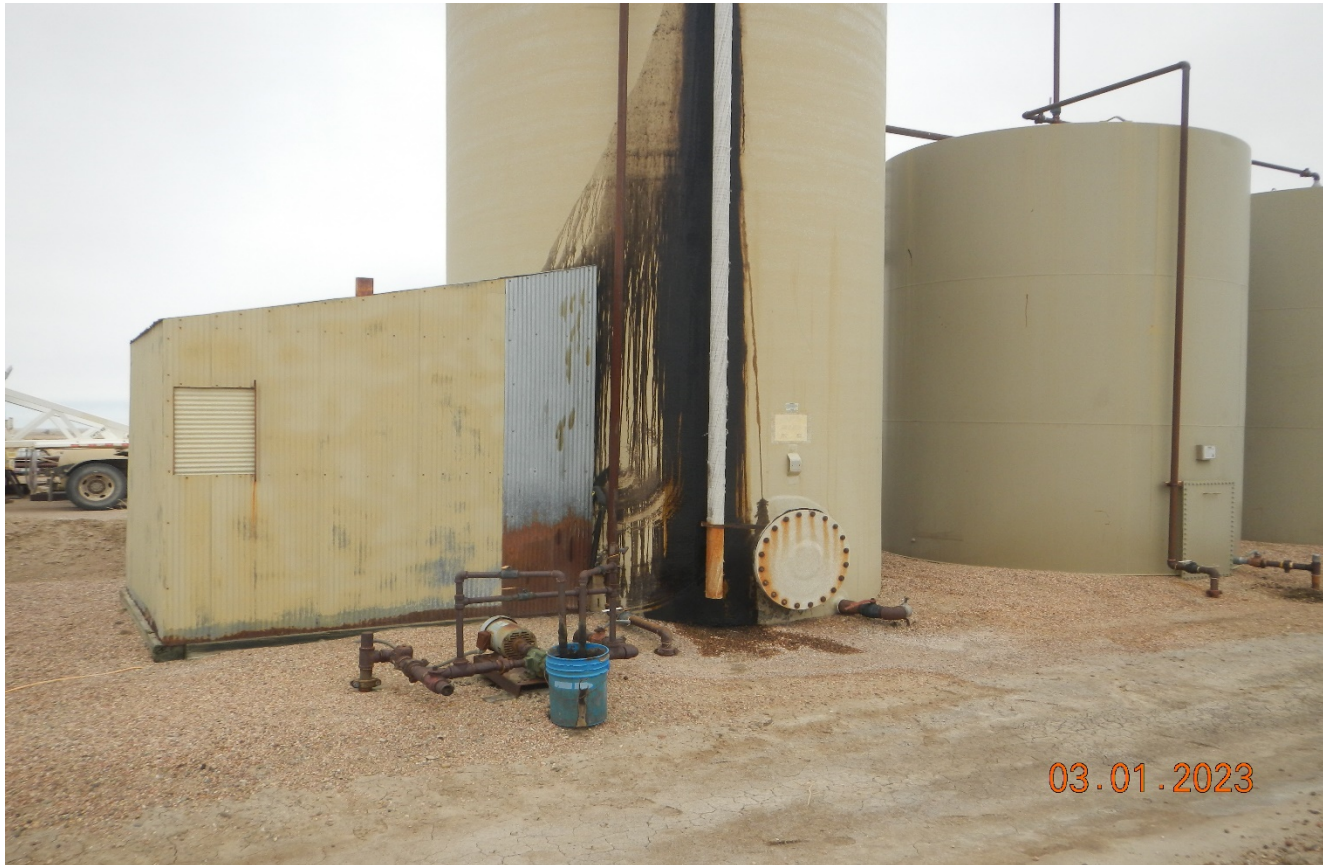
Photo 8. Facing at the back side of the tank battery. There was a spill from the tank which needs to be cleaned up. The blue bucket needs to be emptied and disposed of any oil.
