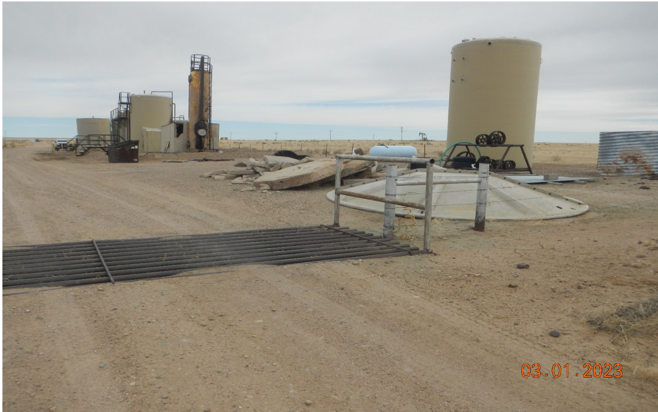
Photo 10. Facing southeast toward the PYLES offsite tank battery and storage yard. There is concrete debris and a broken bottom of a tank among other debris and equipment that must be removed per Rule 606 & 1003.a.
