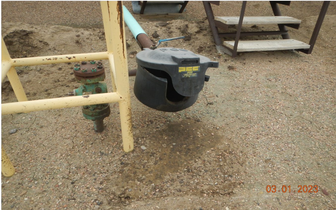
Photo 5. There is oil stained soils at the pipe outlet and oil inside the plastic containment that needs to be cleaned up.
