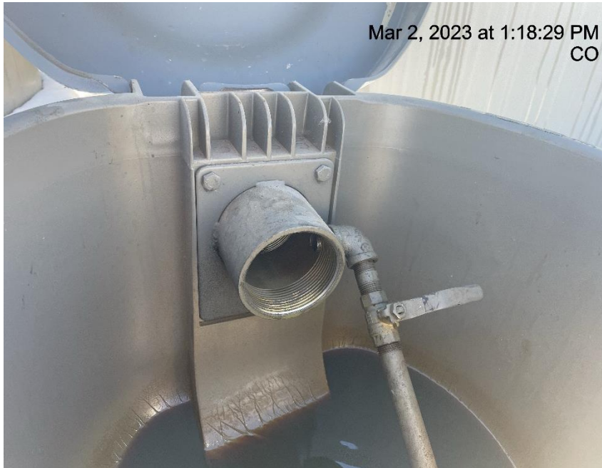
Photo # 1513 Open ended load line
