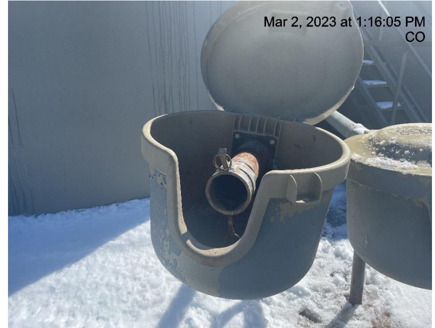
Photo # 1505 Open ended load line
