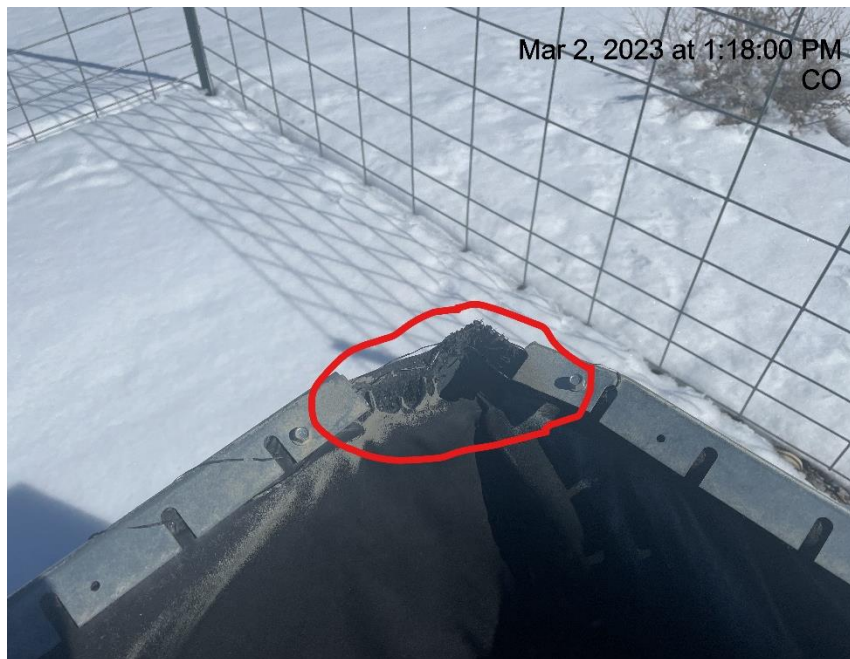
Photo # 1511 Containment needs maintenance
