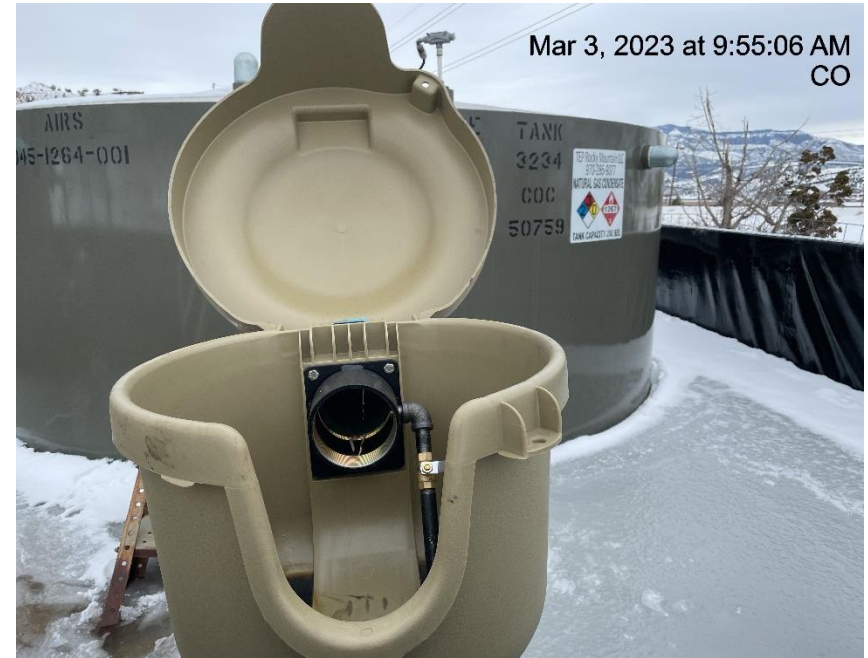
Photo # 1583 Open ended load line
