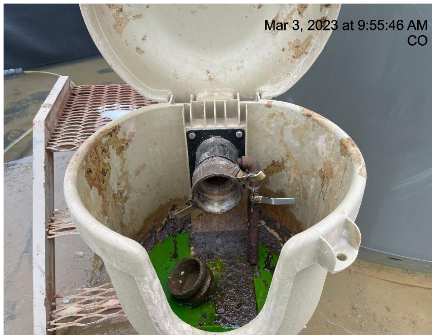
Photo # 1584 Open ended load line
