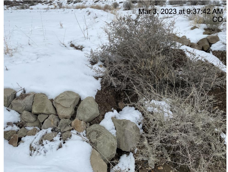
Photo # 1574 Sediment Trap needs maintenance
