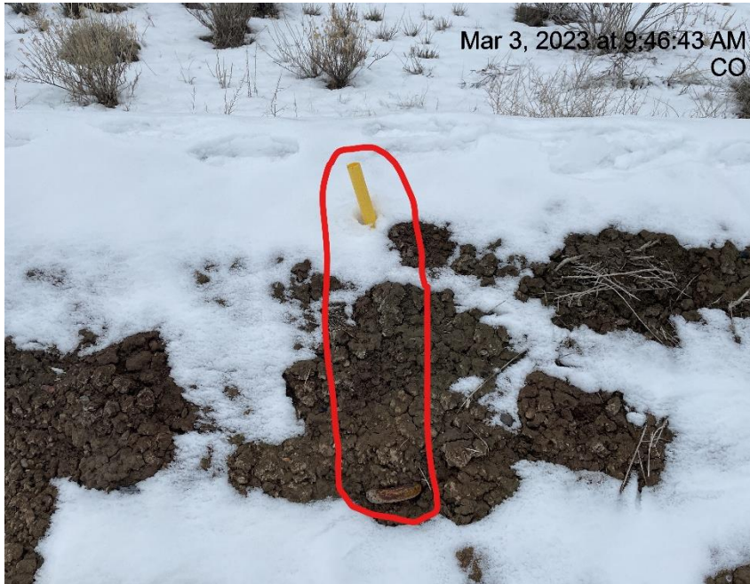
Photo # 1579 Deadman improperly marked
