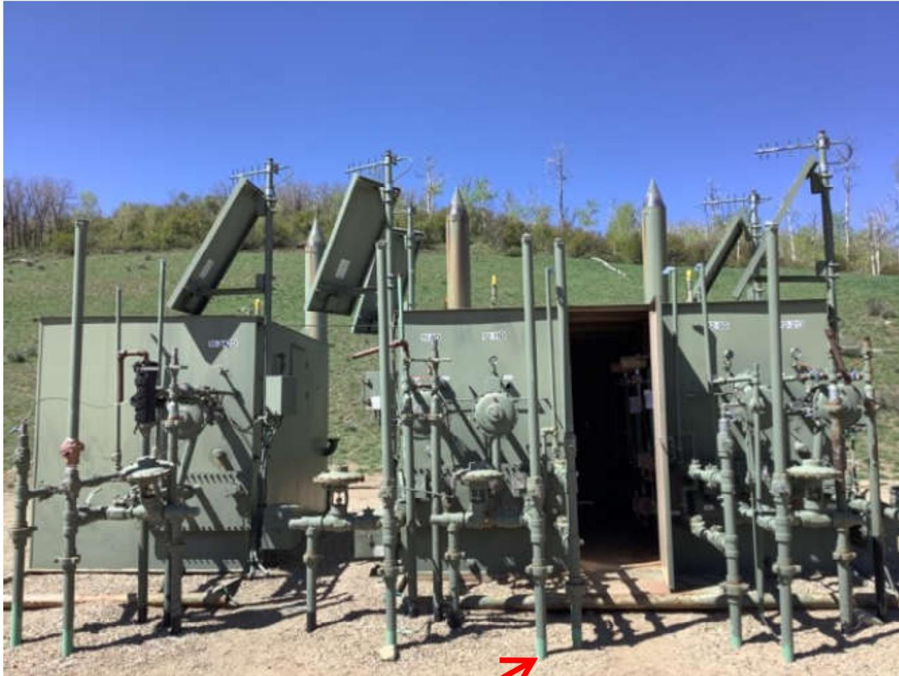
CLOSURE SAMPLE TO BE COLLECTED FROM THE SOIL AT A DEPTH THAT IS BELOW THE NINETY DEGREE ELBOW ASSOCIATED WITH THIS SEPARATOR'S FLOWLINE (WELLHEAD LINE) ATTACHED TO THE 10-4B WELL
