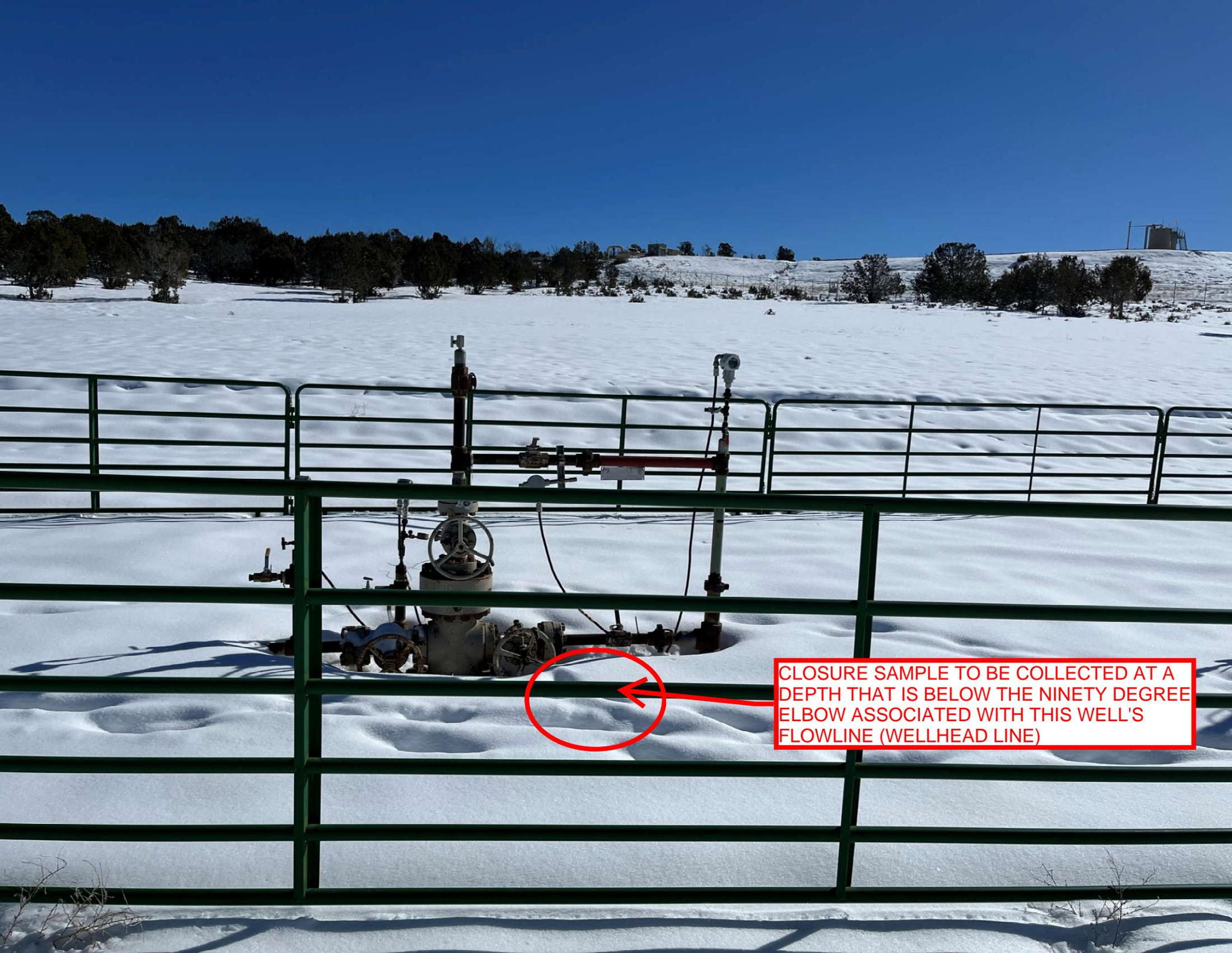
CLOSURE SAMPLE TO BE COLLECTED AT A DEPTH THAT IS BELOW THE NINETY DEGREE ELBOW ASSOCIATED WITH THIS WELL'S FLOWLINE (WELLHEAD LINE)
