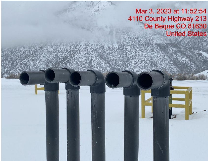
Lack of Wildlife Protection Equipment – Photo #01180
