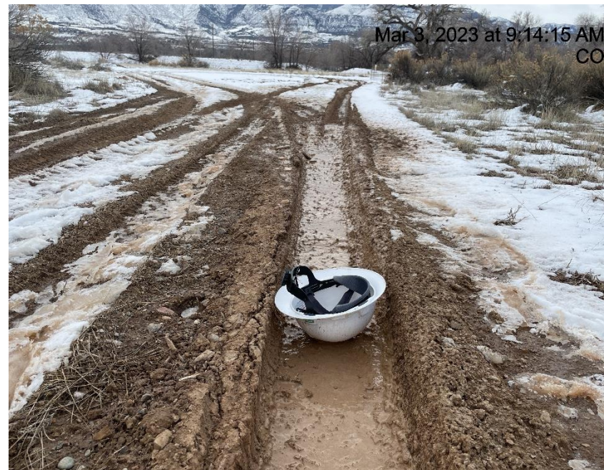
Photo # 1560 Lack of stabilization
