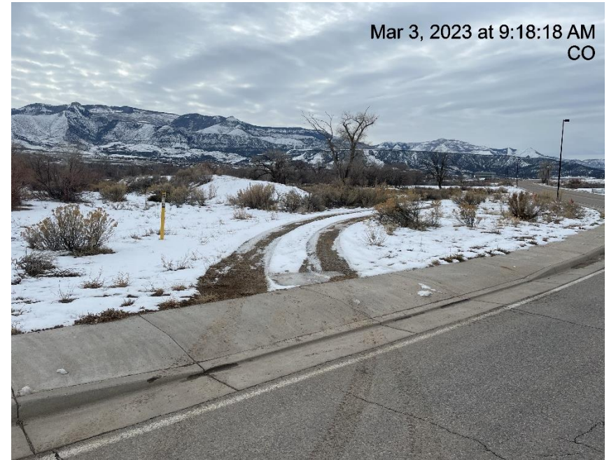
Photo # 1567 Insufficient Tracking BMP
