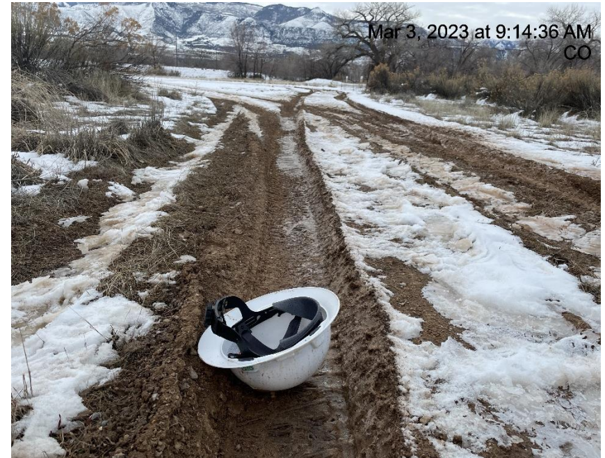
Photo # 1561 Lack of stabilization
