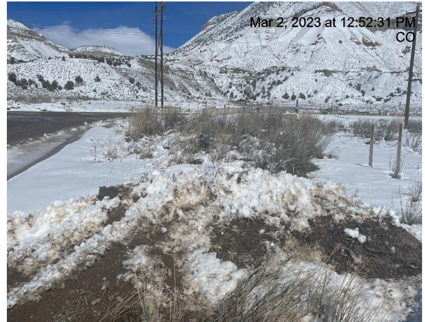
Photo # 1489 Transport of sediment & degradation of vegetation
