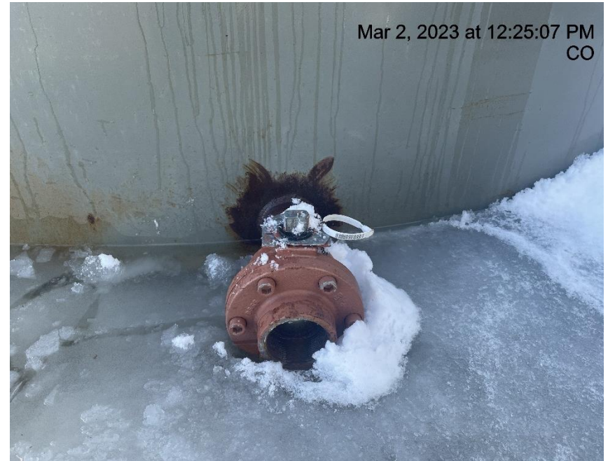
Photo # 1471 Open ended load line
