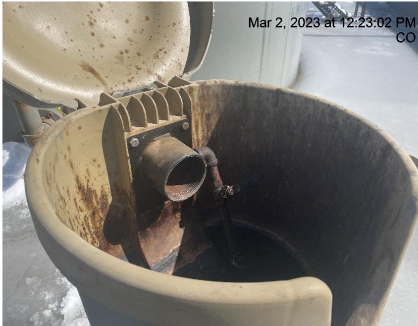
Photo # 1468 Open ended load line
