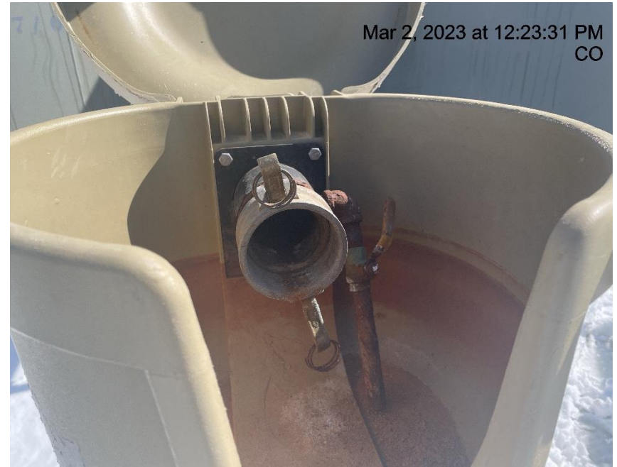
Photo # 1469 Open ended load line
