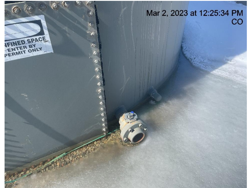
Photo # 1473 Open ended load line
