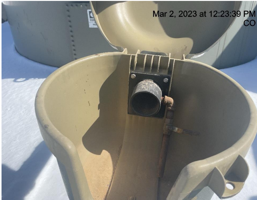
Photo # 1470 Open ended load line
