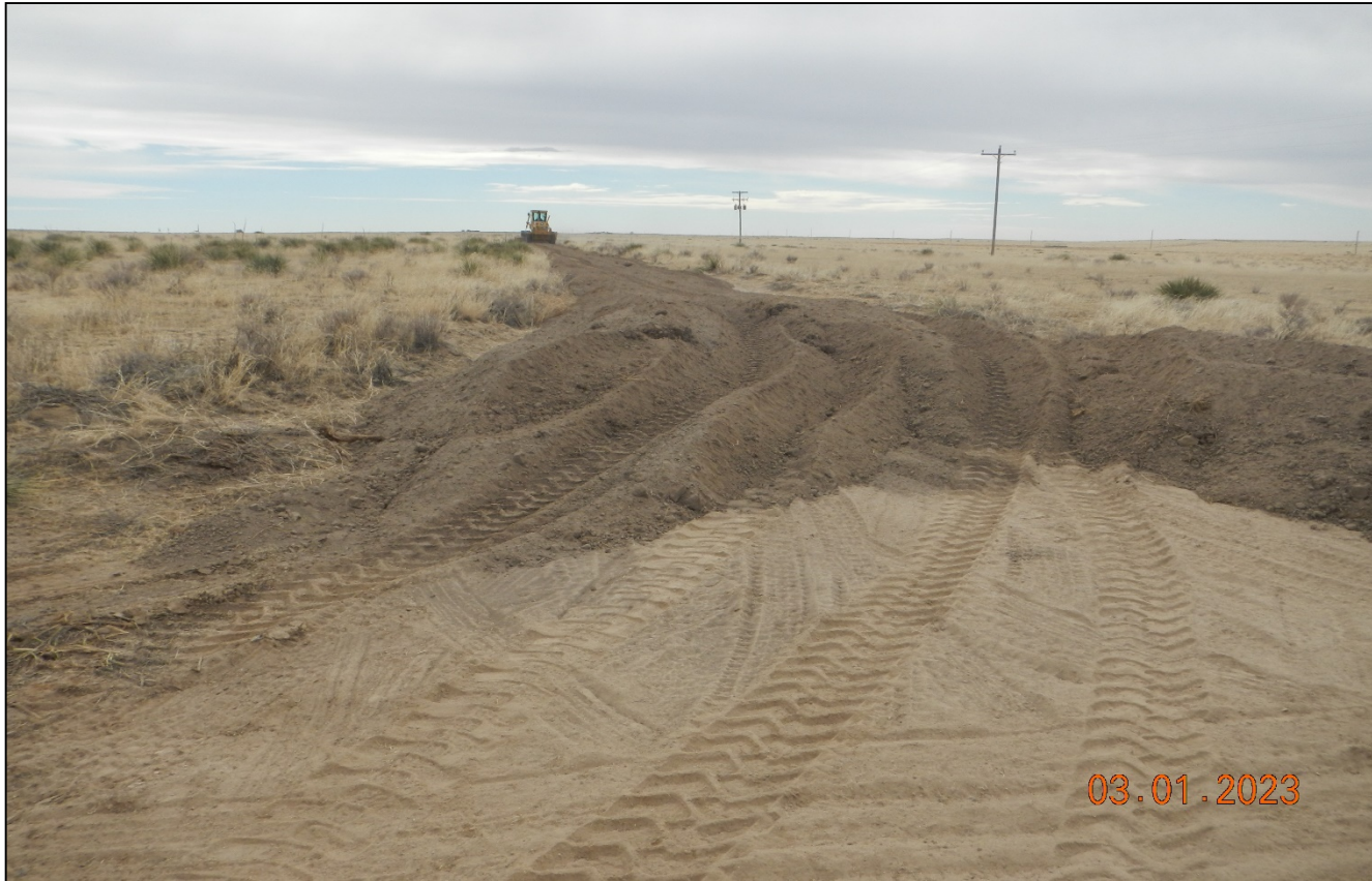
Photo 1. Facing south toward the access road. Topsoil is being hauled in for recontouring of the road.
