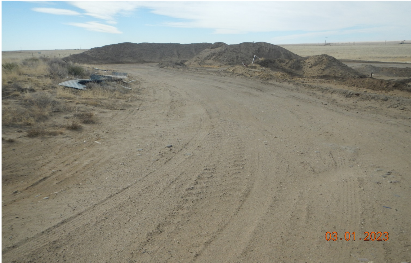
Photo 1. Facing southwest at the DAWSON A 1 tank battery facility. The tank was removed and soils have been excavated in this area. Remediation project: 20712
