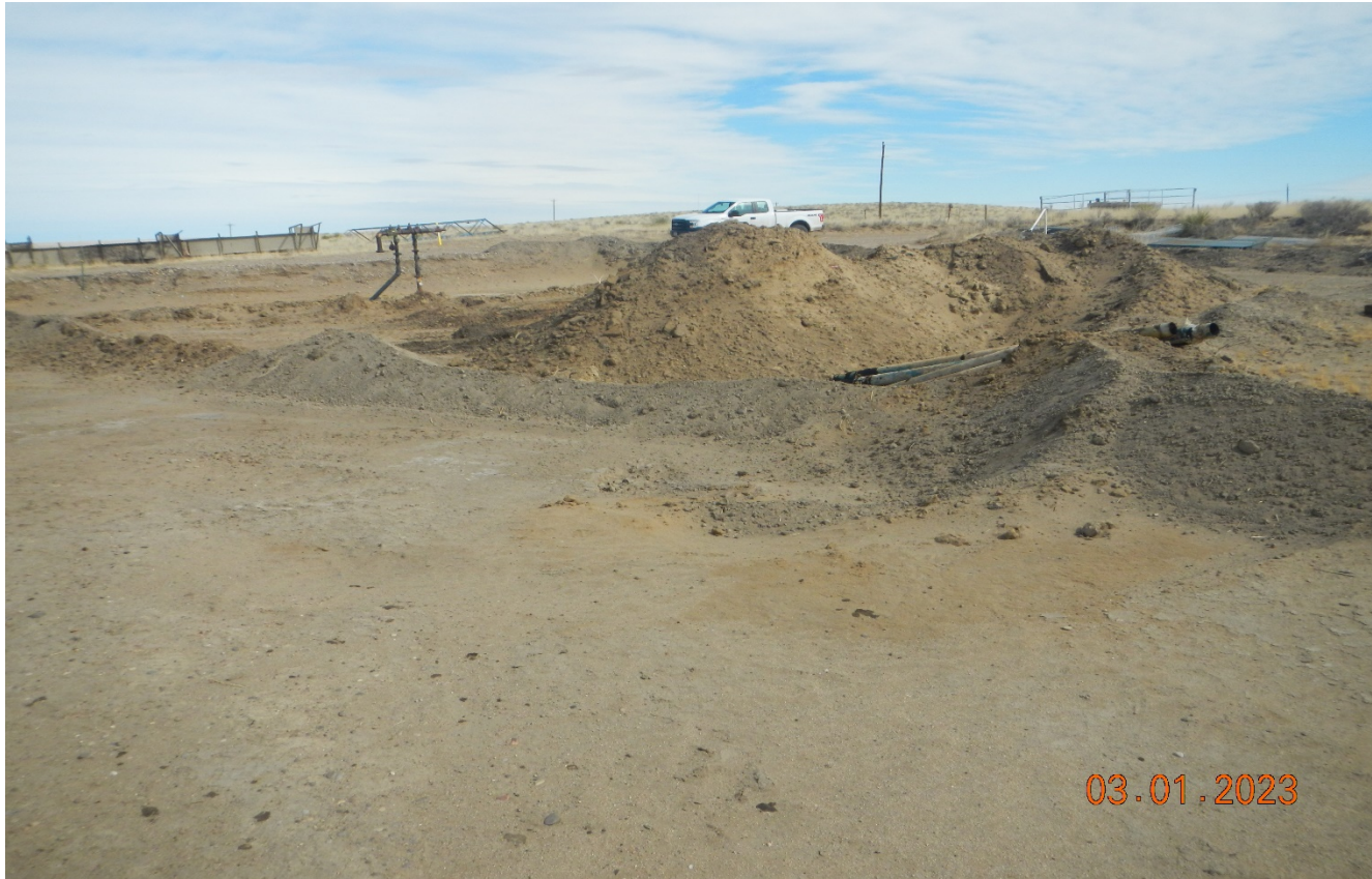
Photo 5. Facing northwest toward tank battery facility. There is loose material being stored that is not stabilized and susceptible to erosion. The berms around the material are not adequately sized or compacted.
