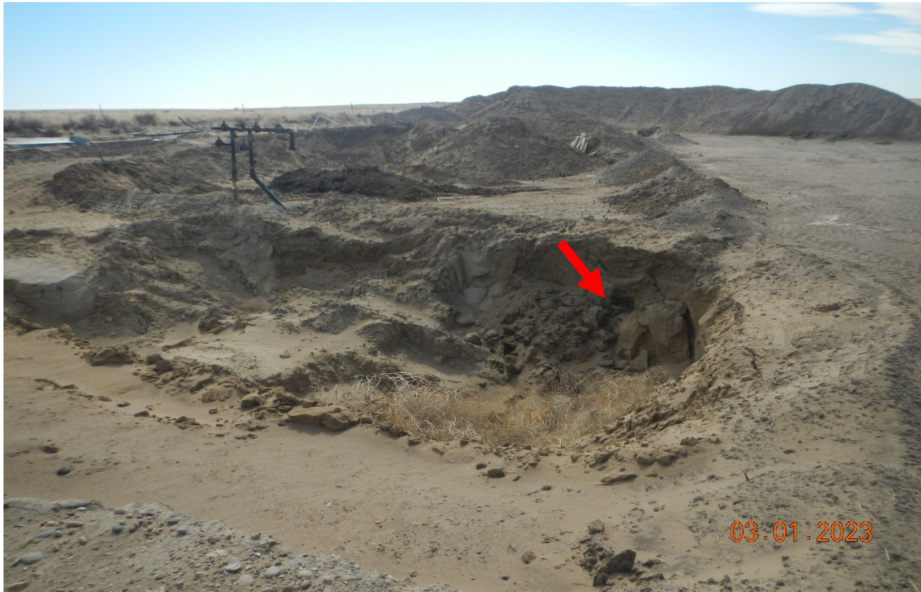
Photo 3. Facing south toward the tank battery facility. The tank was removed and soils have been excavated in this area. There are still oil impacted soil in the excavated area shown at red arrow.
