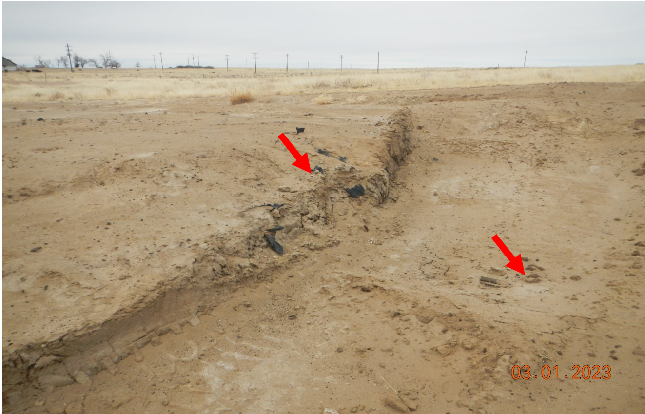
Photo 9. Facing southwest toward the area where the spill occurred. Remediation project: 20712. Some areas have been excavated more than other areas. There are still areas of impacted soils observed. Red arrow points to liner material and stained soil.
