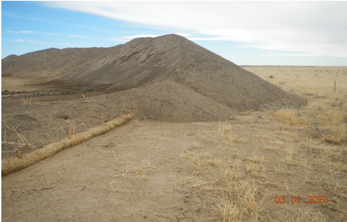
Photo 7. There have been soils brought in and stockpiled at the south side of the location. There is inadequate stormwater BMP's to prevent erosion of the stock piled soil. The wattles have been covered over with soil and are insufficient.
