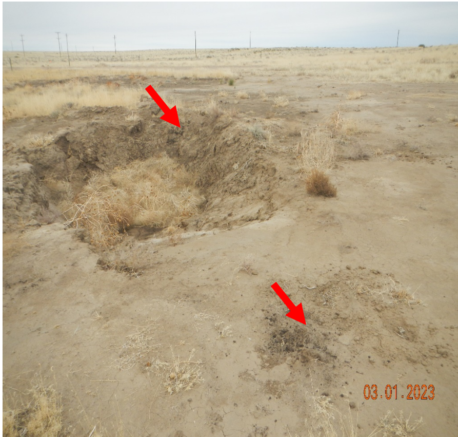
Photo 10. Located at the western side of the spill area. There is an excavated hole at this area approximately 12'x12'6'. There are still areas of oil stained soils at the surface (Bottom left) and 2ft. Down into the excavation area (right photo). Further excavation is needed.
