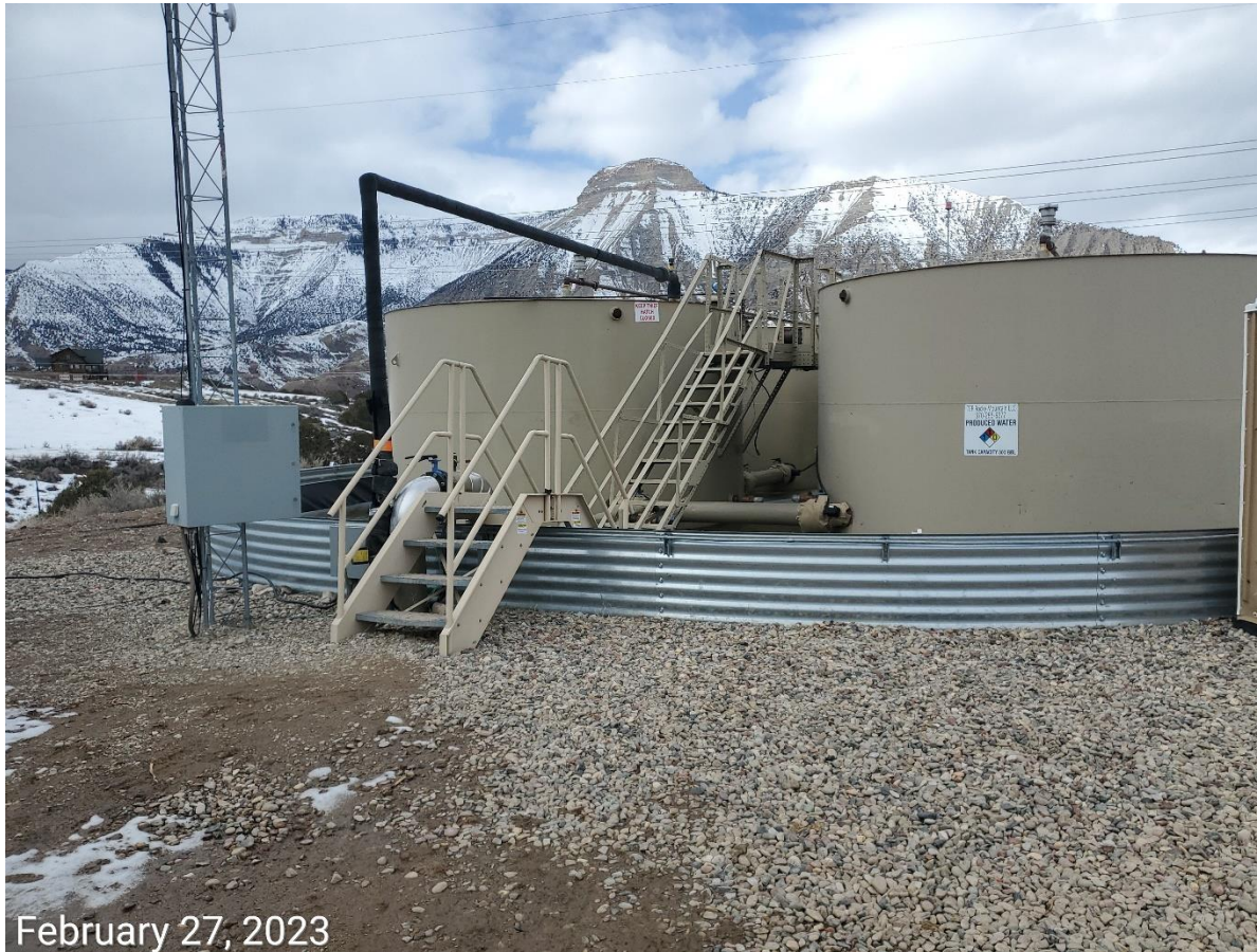
Photo 5: Tank battery on the NW end of the Location. Battery missing signage per 605.e.
