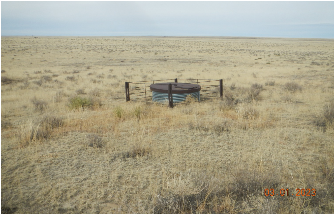
Photo 2. There is a metal cellar that remains at the location which needs to be removed.
