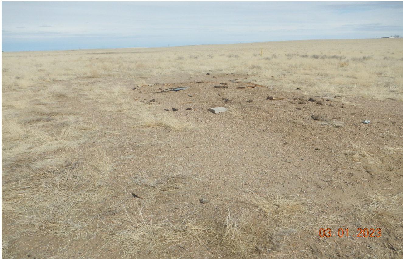
Photo 1. Facing north toward the abandoned wellsite. There is gravel and debris that remains which should have been removed within 3 months of abandonment.
