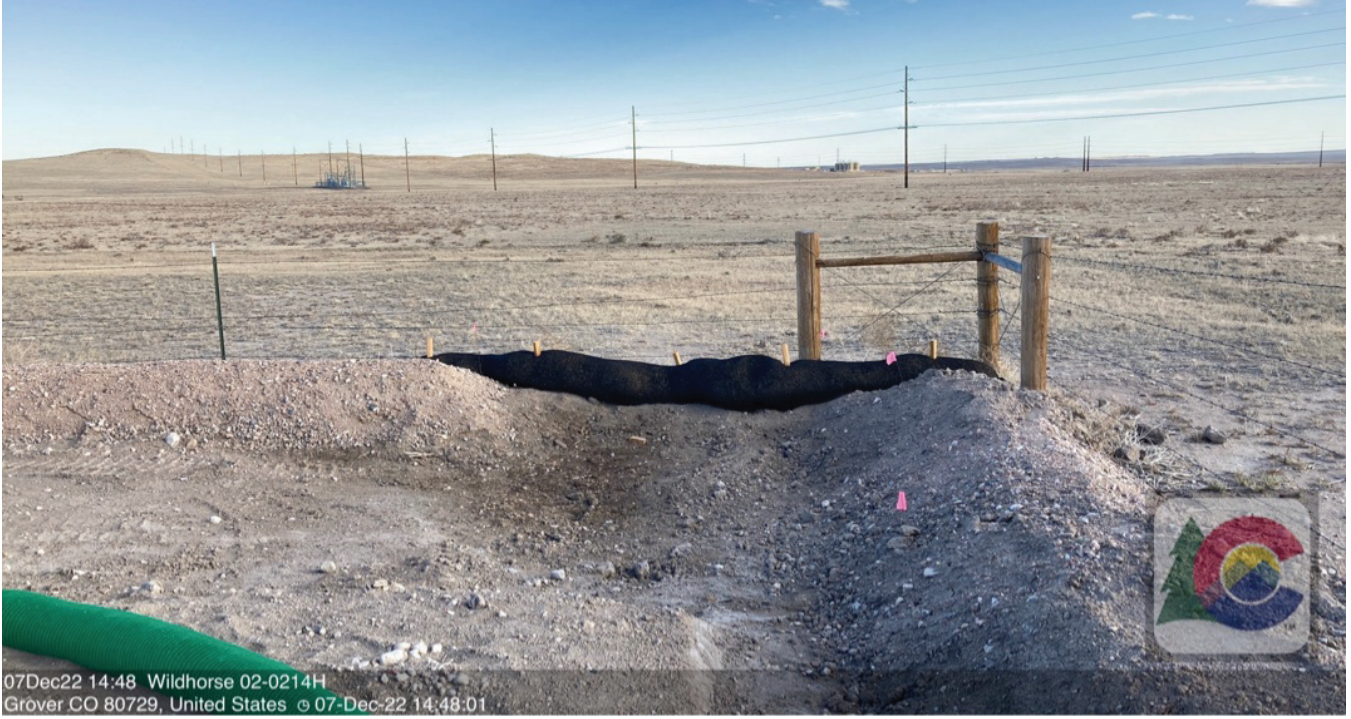
Excavation backfilled and stormwater BMPs improperly installed.
