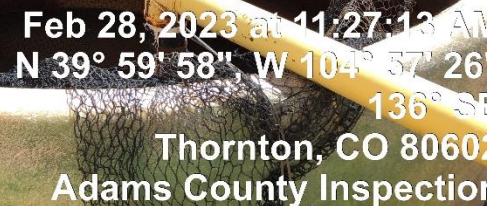
Photo#4 Netting on produced water tank in disrepair
