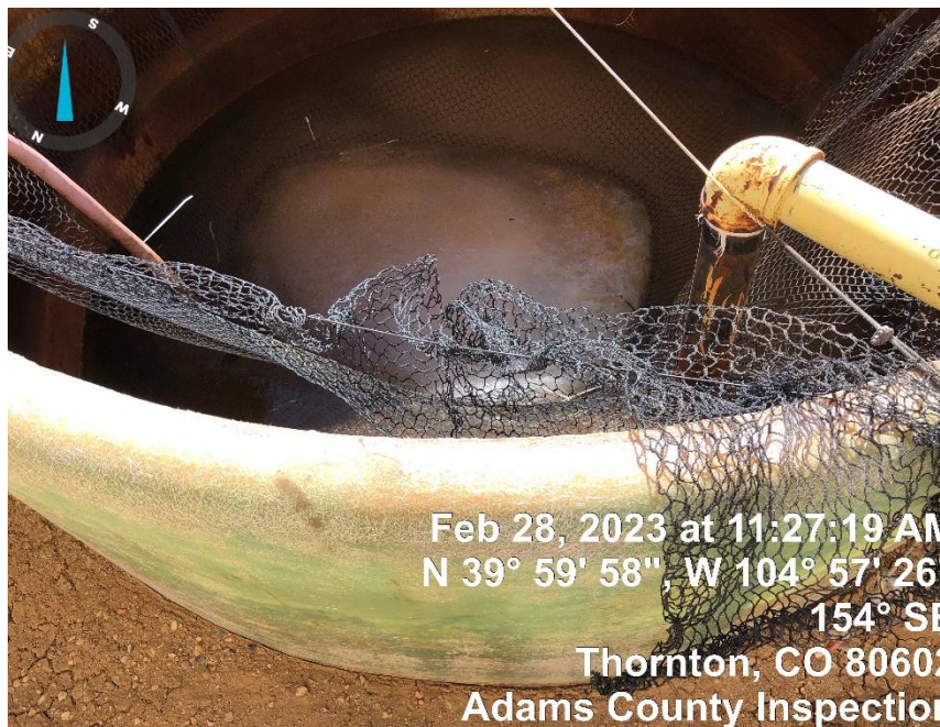
Photo#5 Netting on produced water tank in disrepair
