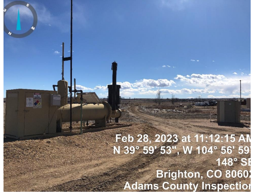
Photo#2 Separator/Gas Meter
