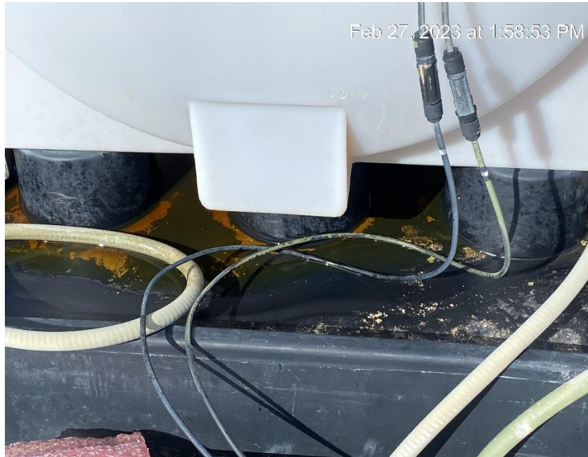
Inadequate fluid level inside containment
