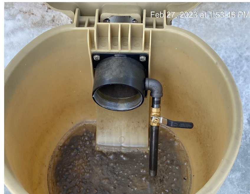
Open end loadline at single tank battery
