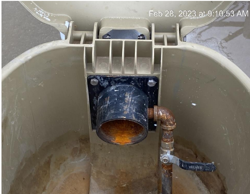
Open end loadline at main tank battery
