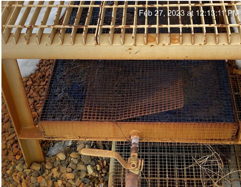
Chemical pump trough full
