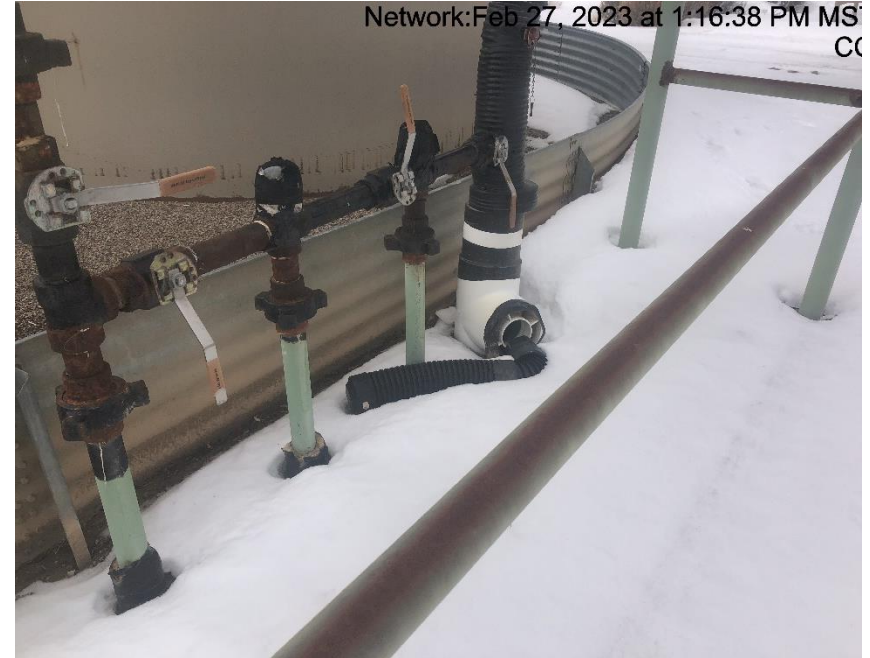
Photo #9098 Flow line heating insulation open ended.
