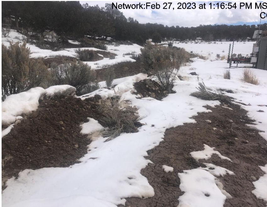
Photo #9099 Sediment has been transported off location and is now choking of vegetation.
