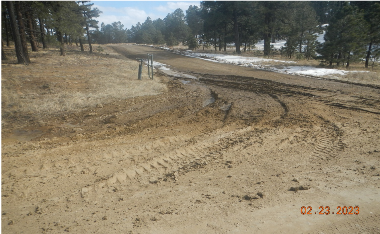
Photo 2. Facing southeast. Drainage from the road shown in the previous photo concentrates at this access road which does not have a culvert. Lat/Long:37.01055,-104.89653
