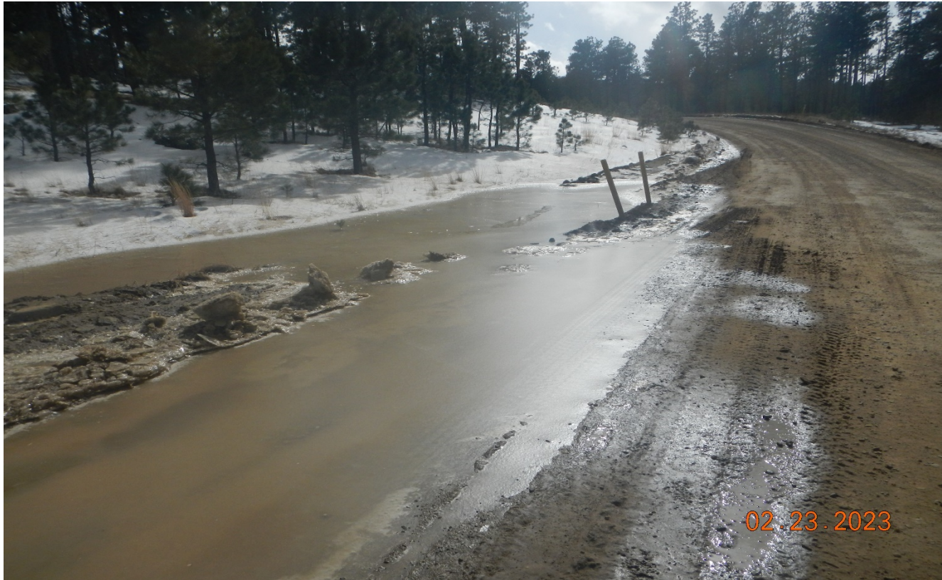
Photo 3. This culvert along the main road may be filled in or iced over and should be cleaned out when it dries out. Lat/Long:37.01149,-104.89621
