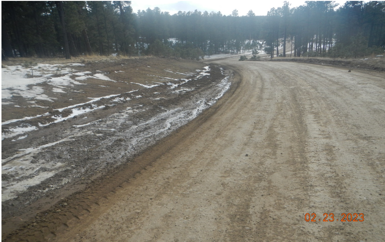
Photo 1. Facing southwest along the main road. The area on the left cut slope of the road should be seeded for stabilization. Lat/Long:37.01249,-104.89533
