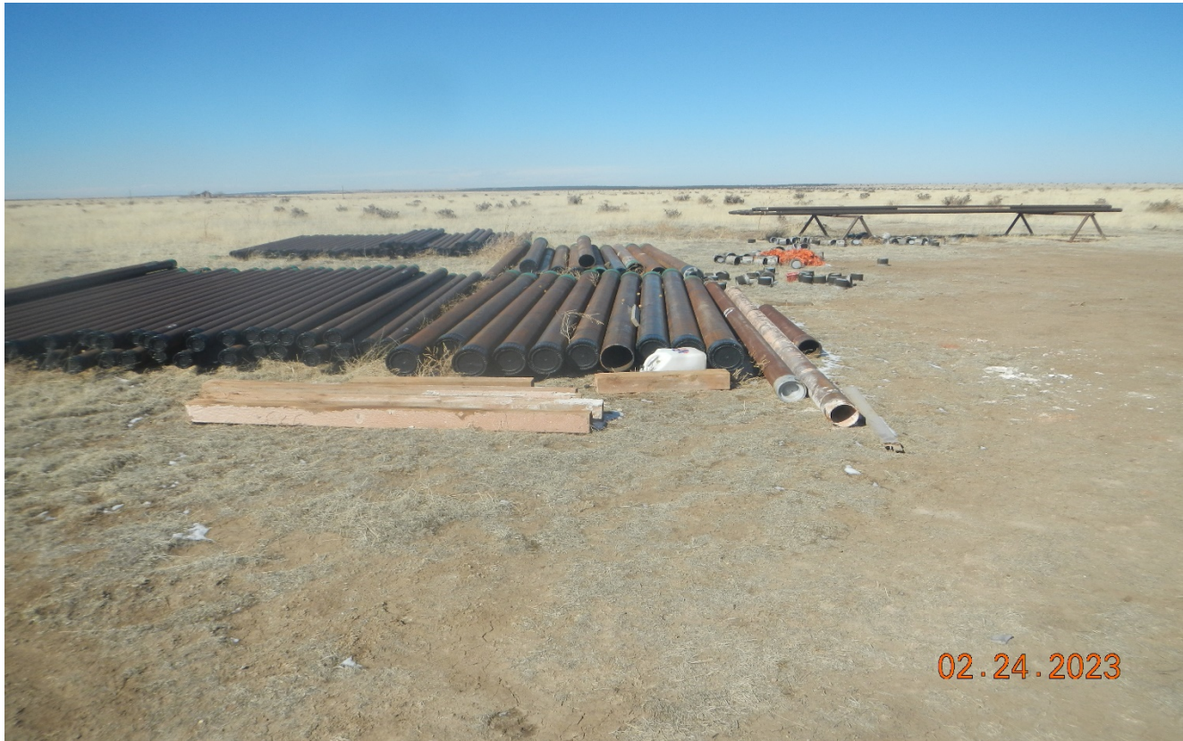
Photo 9. There is drilling pipe and supplies that remain at the southwest side of the location that must be removed.
