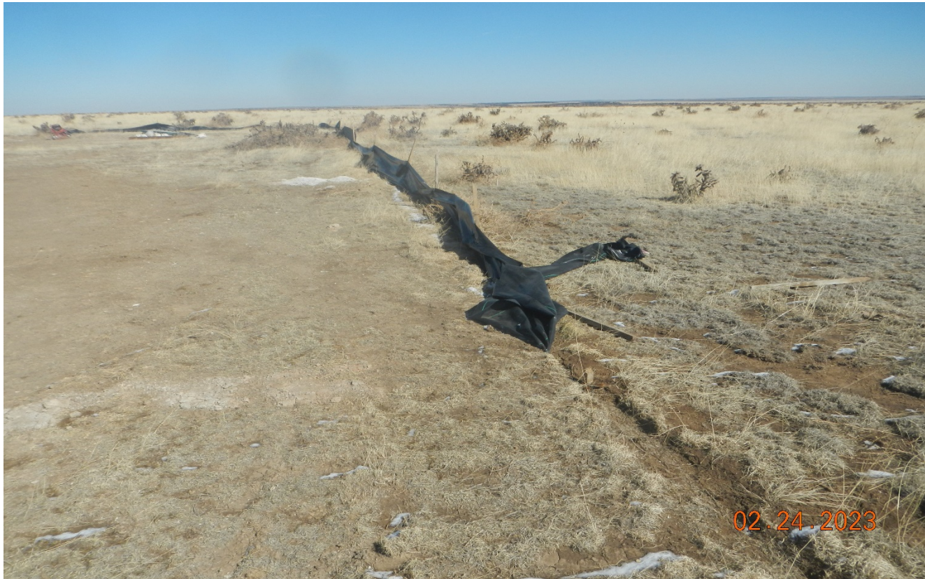
Photo 4. The silt fence is in disrepair. An alternative perimeter BMP may be more appropriate for the location.
