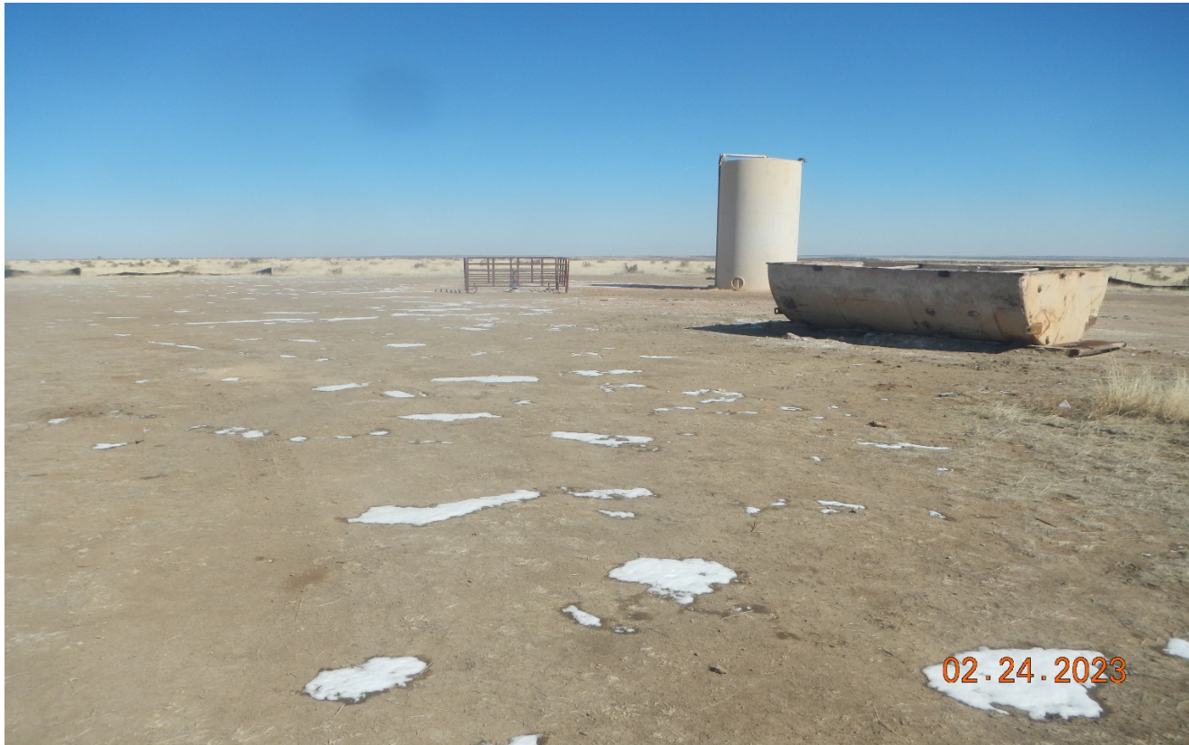
Photo 2. Facing north toward the location. The open top tank is empty and should be removed if unused.
