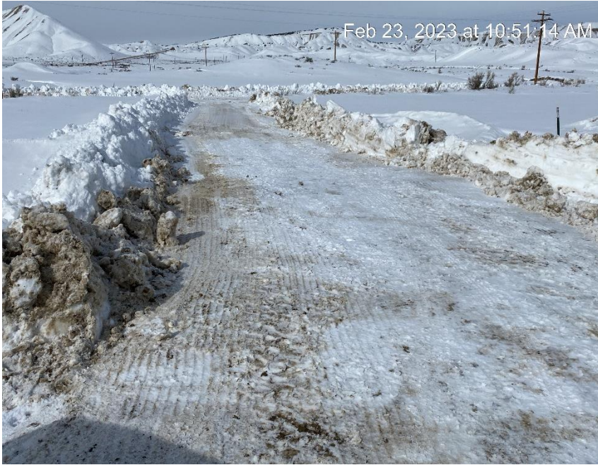
Access road to location
