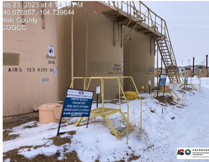
Pic 7 tanks, signs
