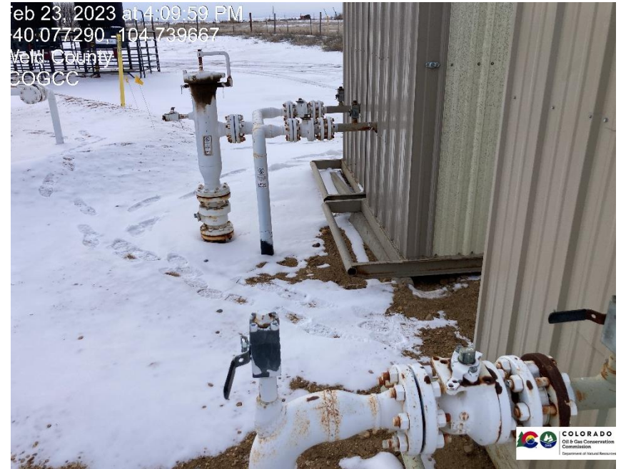
Pic 4 gas meter run valves appear to be open
