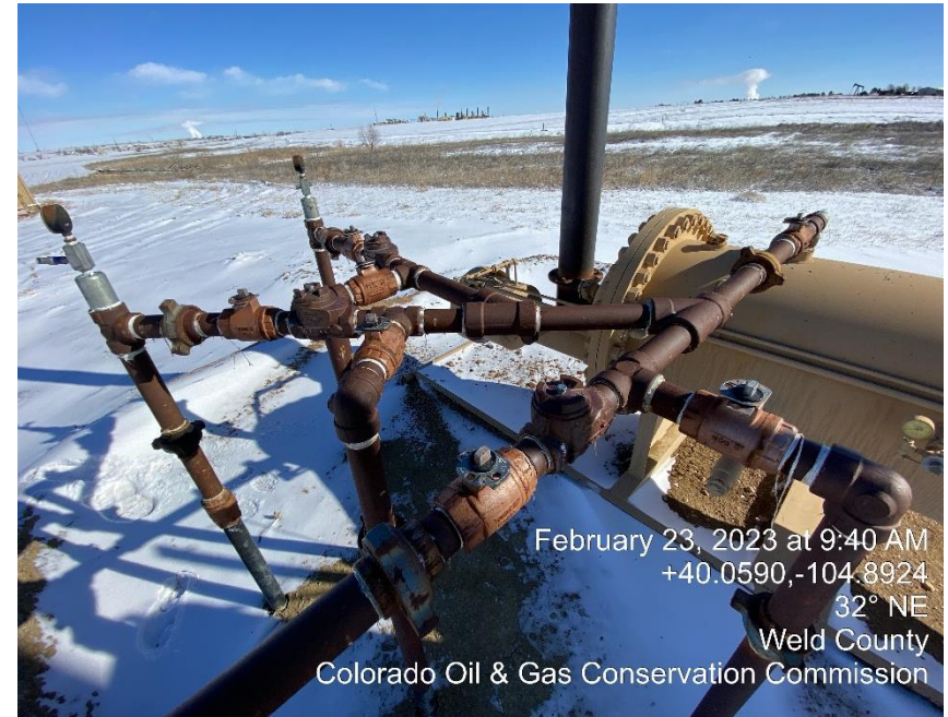
Photo #4 Balon valves appear to be open
