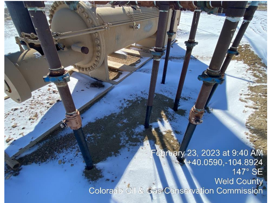
Photo #2 Balon valves appears open
