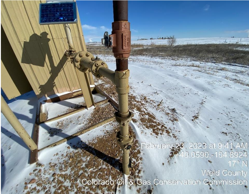
Photo #5 Balon valve on upstream of gas meter run appears to be open
